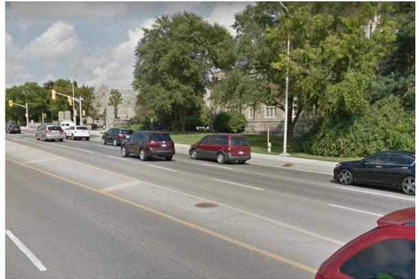
Maintenance holes positioned outside the wheel path of vehicles and bicycles in London.
