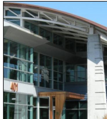
4. Windows designed as glass curtain wall systems (where they are not treated as a separate element from the façade system) should be designed with projecting vertical and/or horizontal mullions, or other modulating features.
