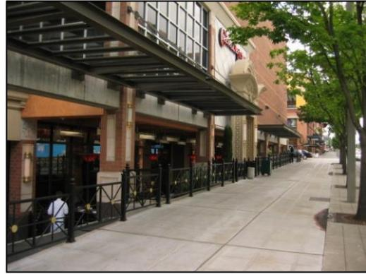
5. Drainage should be designed so that the awning or canopy does not drip on pedestrians.
