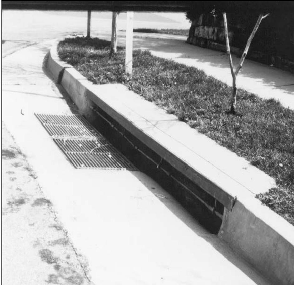
**Figure 4-16. Sweeper combination inlet.**
