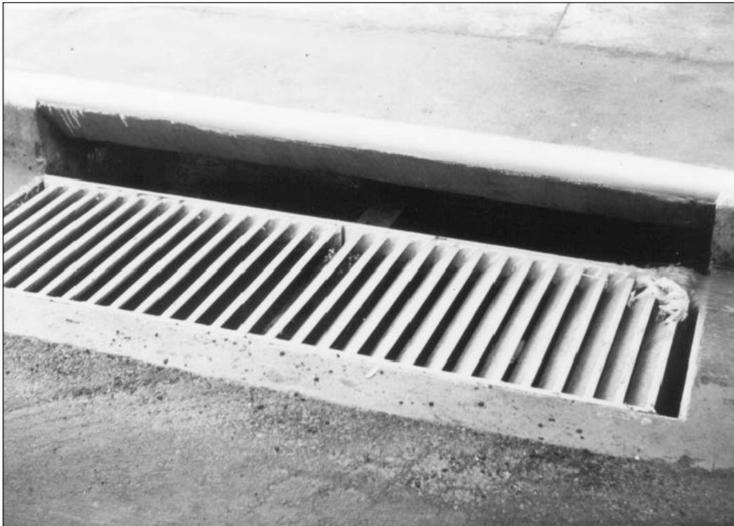
**Figure 4-15. Combination curb-opening, 45 degree tilt-bar grate inlet.**
