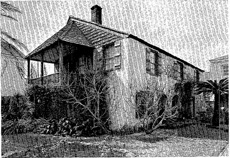
12A Garden Facade, Oldest House
