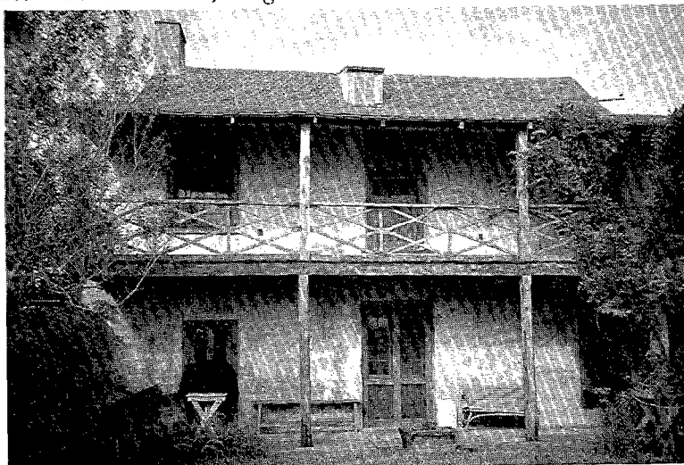
19B Garden Facade, Long-Sánchez House
