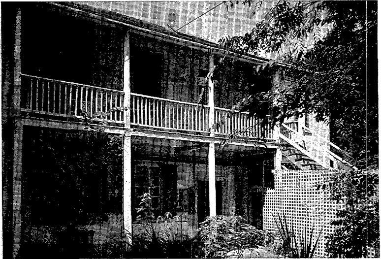
24B Garden Facade, Poujoud-Slater House
