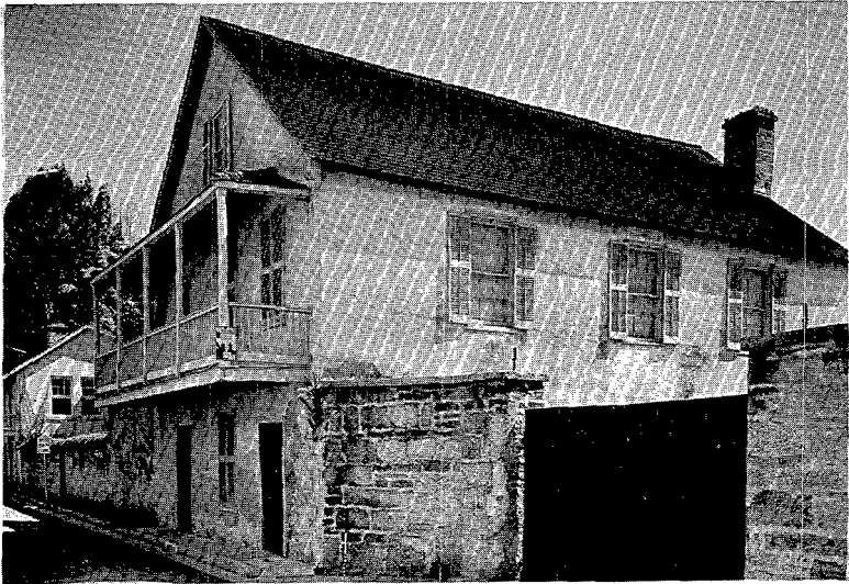
16A Street Facade, Don Miguel de O'Reilly House, Aviles Street
