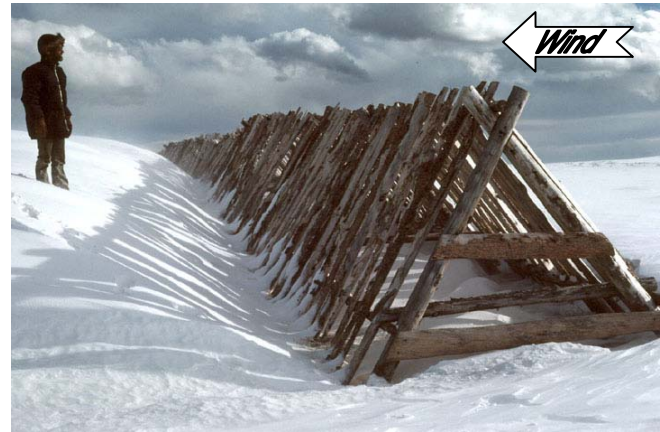
Figure 6.19. Vertical slats attached to buck-and-pole supports (Tabler 1986b).
