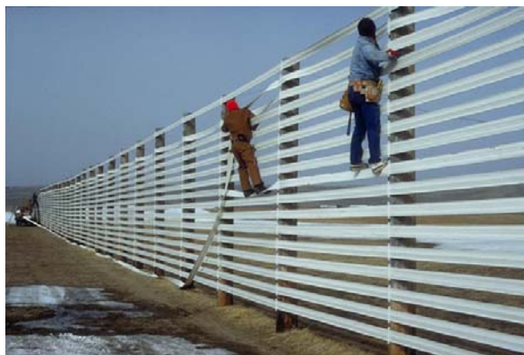
Figure 5.29. Composite polyethylene / stranded steel wire fencing material (Centaur HTP ® ). Lower right photo courtesy of Perma-Rail ® International. (Upper left from Tabler 1994).
