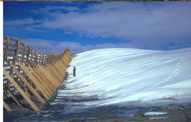
Figure 2.9. Snow accumulation at Wyoming I-80 Mile 269.5 in 1970 before fencing (upper left), compared with conditions typical of the 31 years since fences have been installed (right). The lower view shows a 3.8-m (12.4-ft) Wyoming fence with snow accumulation on the same date at another location. (From Tabler 1973a).
