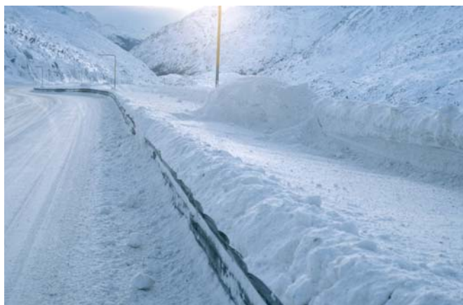
Figure 5.15. Safety barrier prevents removal of roadside snowbanks.
