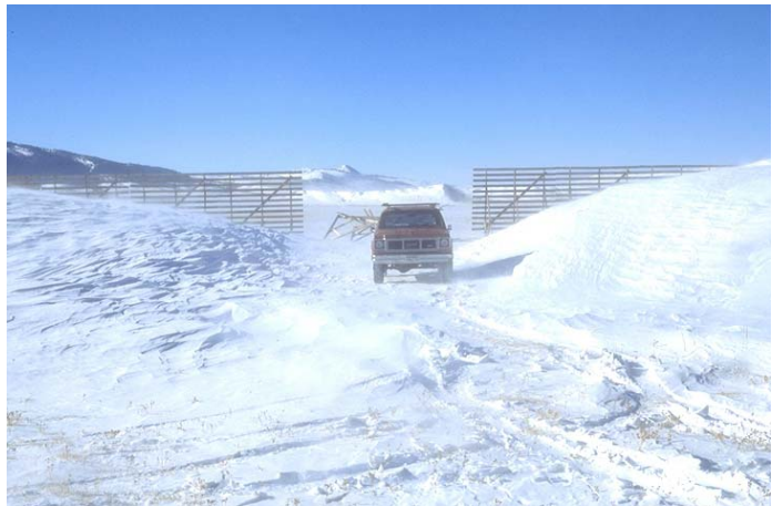
Figure 6.85. Opening in fence suitable for year-round off-road access (Type B, Figure 6.83). Fence height is 4.3 m (14 ft).
