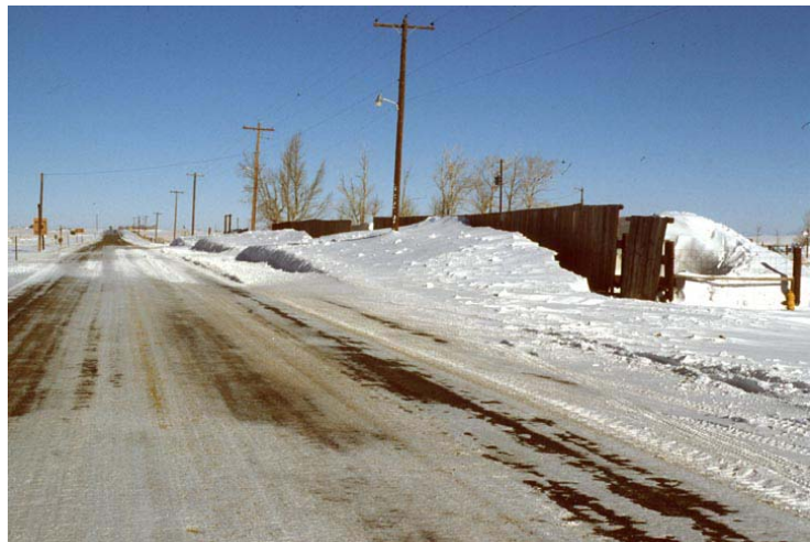
Figure 4.4. A board fence, 2.4-m (8 ft) tall, that caused a drift on the road. Wind was from left. Structures and vegetation on the downwind side of the road are sometimes overlooked during summertime field reviews (Tabler 1994).
