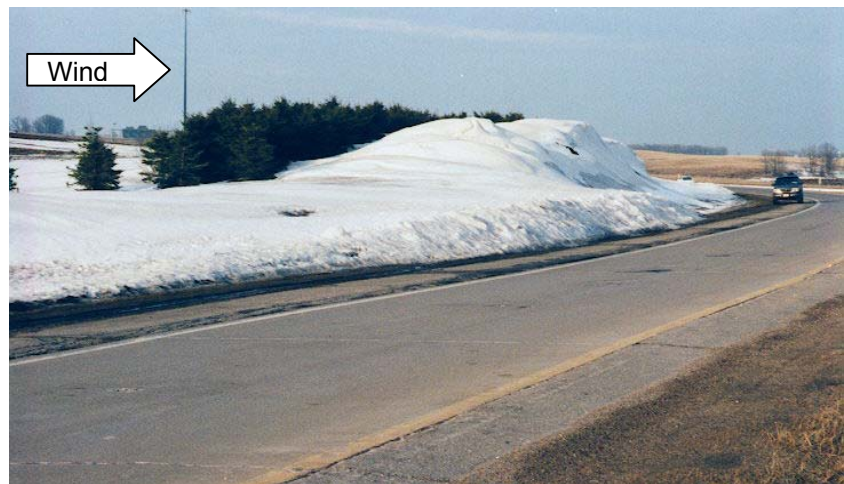
Figure 7.7. Severe drifting problems were caused by an opening in this dense spruce planting.
