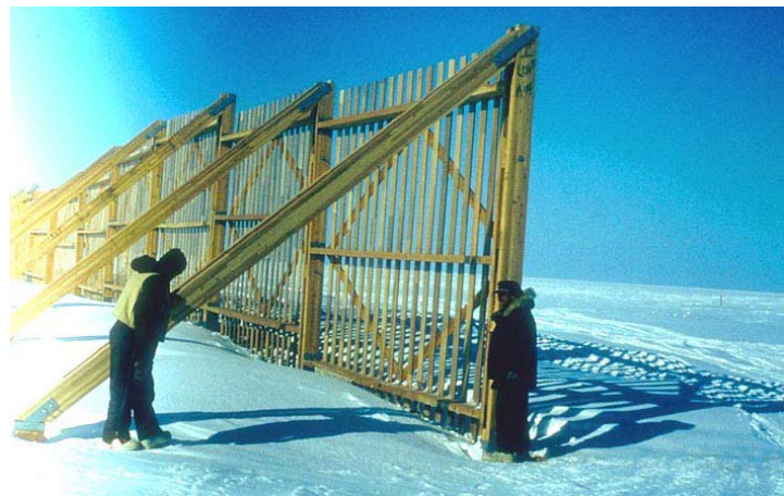
Figure 6.25. Vertical slats supported by horizontal stringers between vertical supports were used for this 4.6-m-tall (15 ft) fence at Wainwright, Alaska (Tabler 1994). Photo by George Clagett, U.S. Soil Conservation Service.
