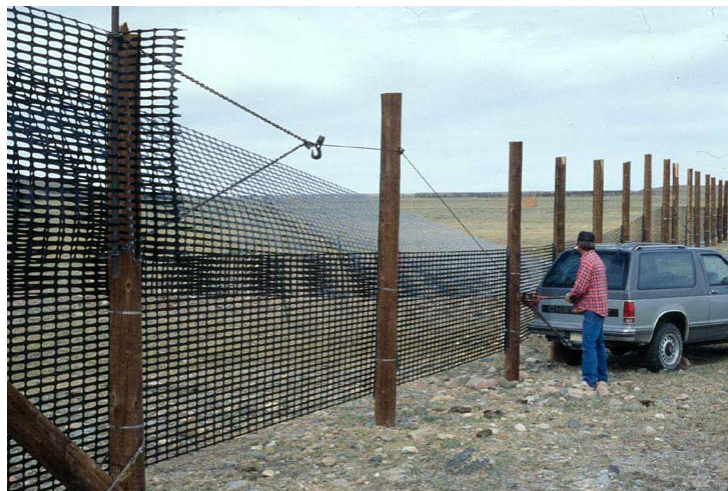
Figure 6.35. A method of tensioning multi-tiered plastic fencing (Tensar® UX3100 snow fence)(Tabler 1994).
