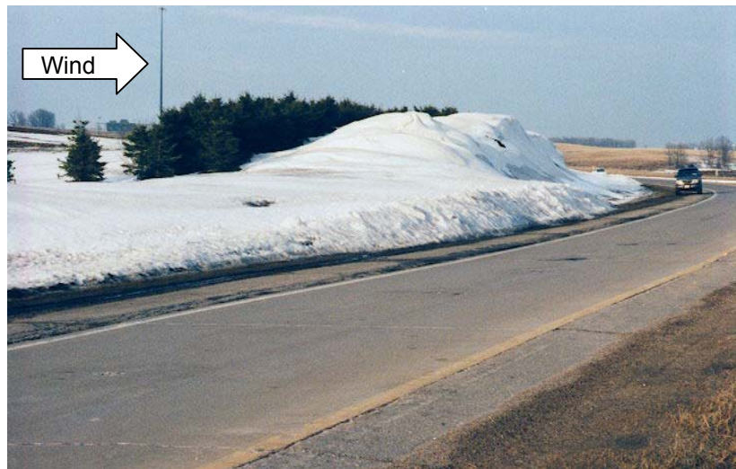
Figure 5.34. Gaps in living snow fences with insufficient setback cause deep drifts on the road.
