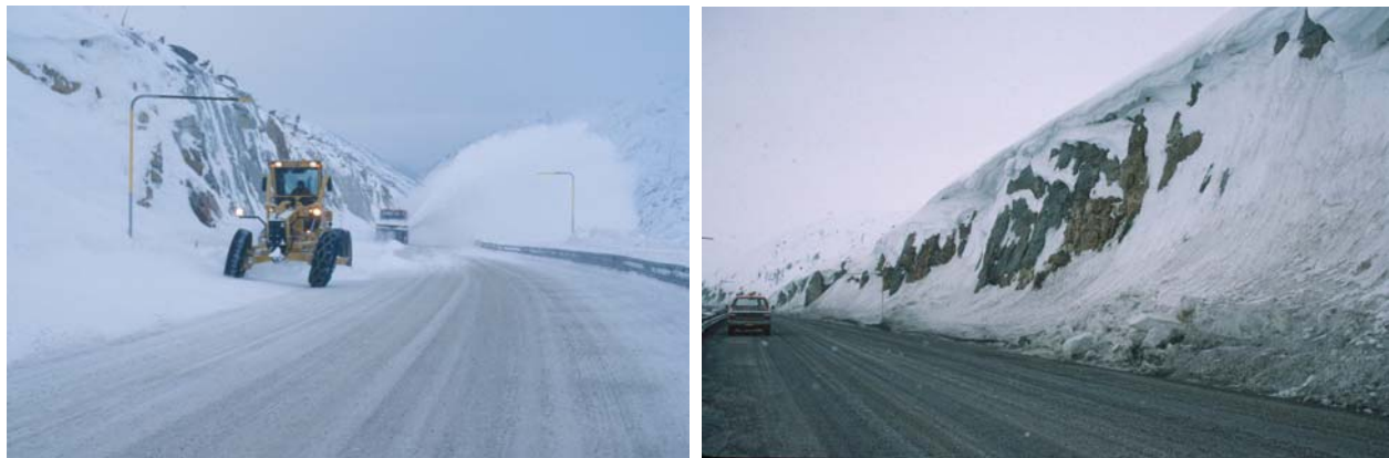
Figure 8.30. The recommended minimum 3.7-m ditch width provides space for snow sloughing and temporary snow storage. These examples on the Klondike Highway illustrate snow problems associated with a narrow ditch.
