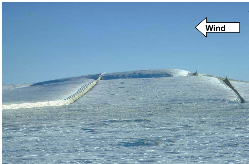
Figure 6.77. Wind blowing up-hill toward a 1.8-m-tall (6-ft) fence caused a "super-drift" that buried the second 3-m-tall (10 ft) fence located 55 m (180 ft) downwind. The drift contained four times as much snow as a 1.8-m-tall fence on flat terrain (Tabler 1986b).
