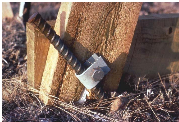
Figure 6.12. It is imperative to tighten the U-clip to prevent slippage. Right view shows rebar that has nearly rasped entirely through bolt and U-clip.
