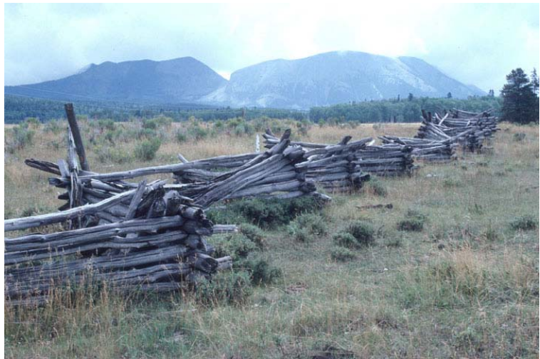
Figure 6.21. Pole crib fence near La Veta Pass, Colorado (Tabler 1986b).
