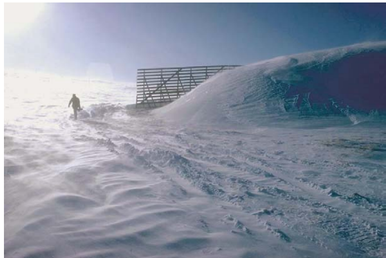
Figure 3.42. Rounding of drift ends, as shown by this 3.8-m-tall (12.4-ft) Wyoming fence, reduces storage capacity and trapping efficiency (Tabler 1986).
