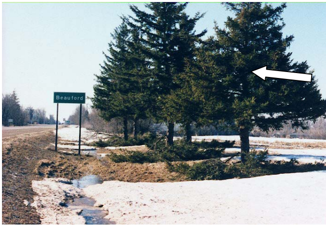
Figure 7.30. Pruning lower branches of roadside trees can mitigate snowdrifts. Pruning the trees in the upper right view would prevent the snowdrift at this location. Arrows indicate wind direction.
