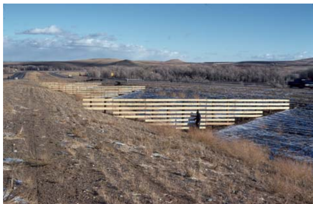
Figure 6.79. Median fences should be spaced 10 times their greatest height (right from Tabler 1994).
