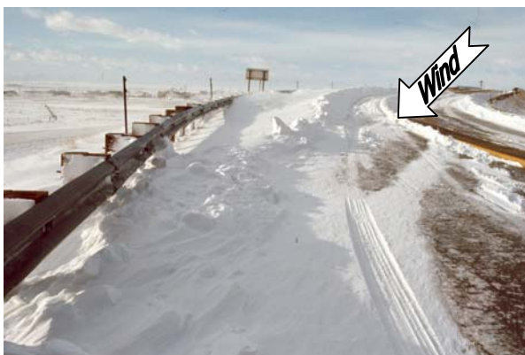
Figure 8.37. W-beam beam safety barrier causes snowdrifts and obstructs plow cast (left from Tabler 1994).
