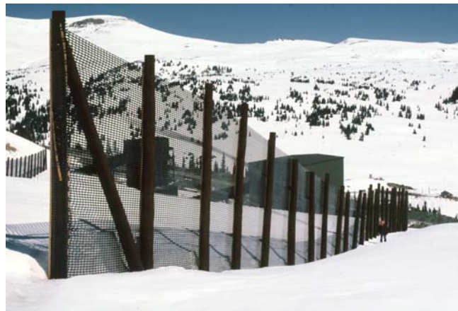
Figure 6.32. End supports must be braced longitudinally for tensioning synthetic materials (Tabler 1994). Tensar® UX3100 material was used for this 5-m (16-ft) tall snow fence at Summitville, Colorado.
