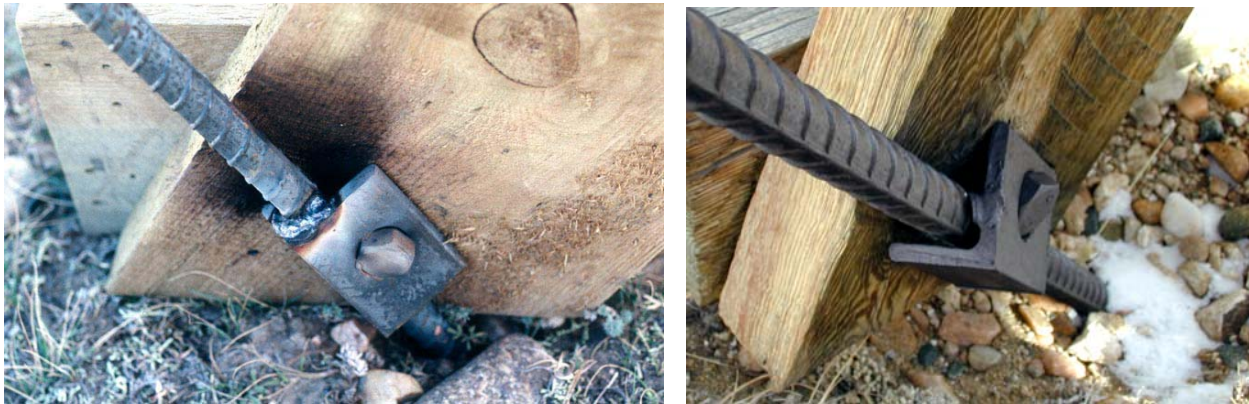
Figure 6.13. Steel angle can be used for anchor attachment, but rebar must be welded to angle to avoid failure after wood dries and shrinks. Vibration has led to failure of the light tack weld in the photo on the right. Left photo from Tabler (1994).
