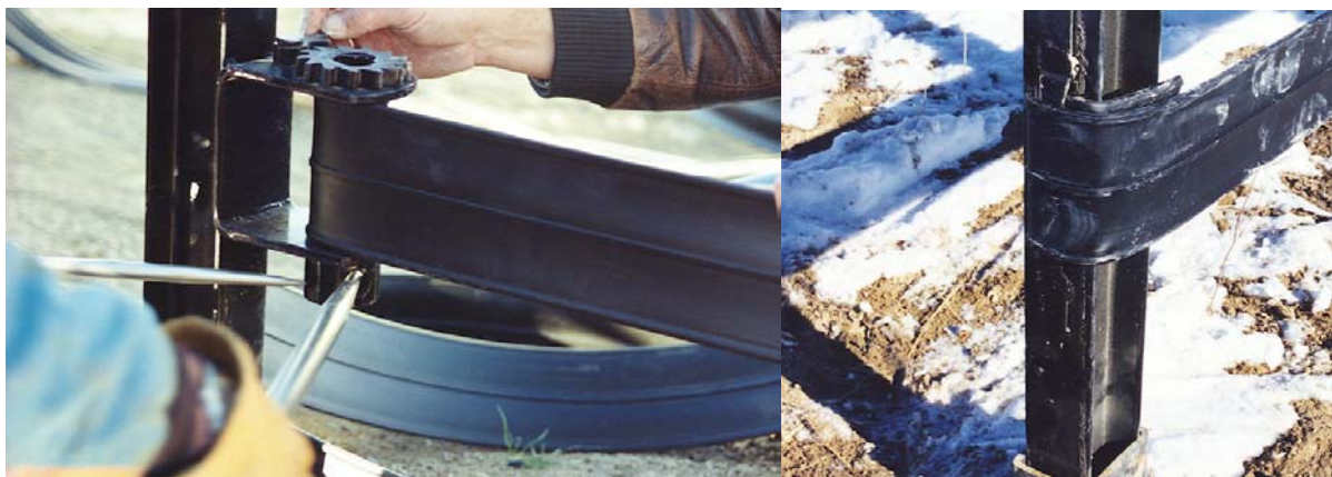
Figure 6.38. Left: Ratchet winch permanently attached to end of fence line facilitates installation and maintenance. Right: Method of attaching "dead" end to post.
