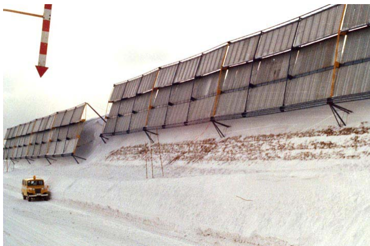
Figure 6.64. The effect of this large deflector on snow deposition is shown in the sketch redrawn from Hokkaido Development Bureau 1974, page 19 (Tabler 1994). Photo by Tetsuya Uchiya, Hokkaido Development Agency.
