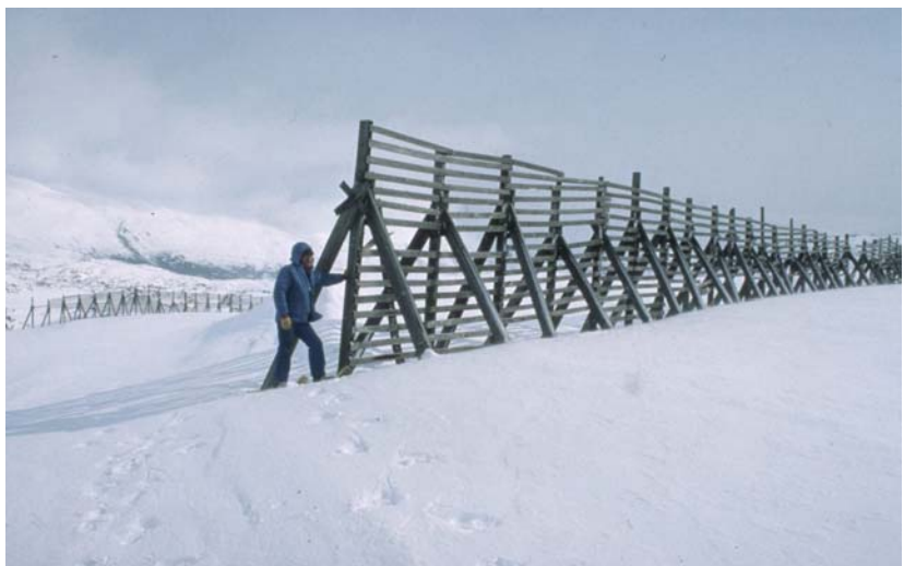
Figure 2.5 Snow fences on the White Pass and Yukon Railroad, approximately 25 km (16 miles) north of Skagway, Alaska (Tabler 1994). Built in 1900, they were 4 m tall (13.5 ft).
