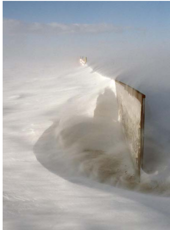
Figure 3.60. Snow particles jetting over the top of a solid barrier 1.2 m (4 ft) tall illustrate why the trapping efficiency declines after the upwind drift reaches the top of the fence (Tabler 1994).
