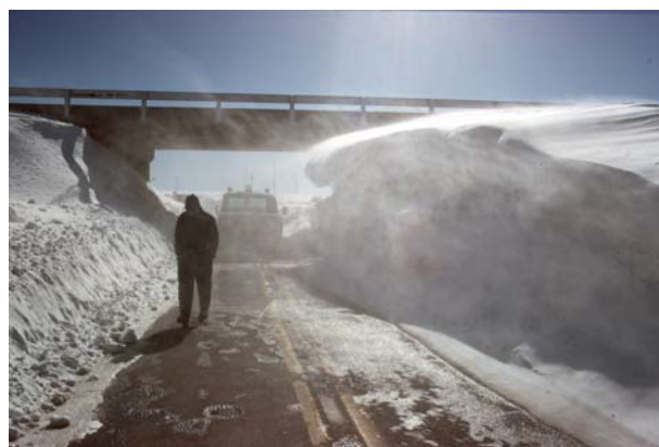
Figure 7.20. Typical snowdrift problem associated with grade separations.
