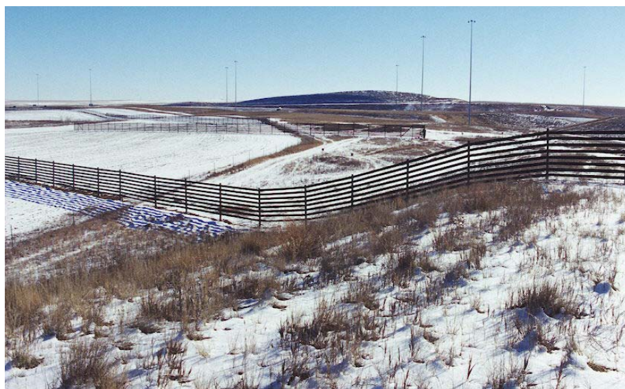
Figure 6.45. Composite rail accommodates irregular terrain, but posts at low spots must be properly anchored to resist the upward force generated by the tensioned rails.
