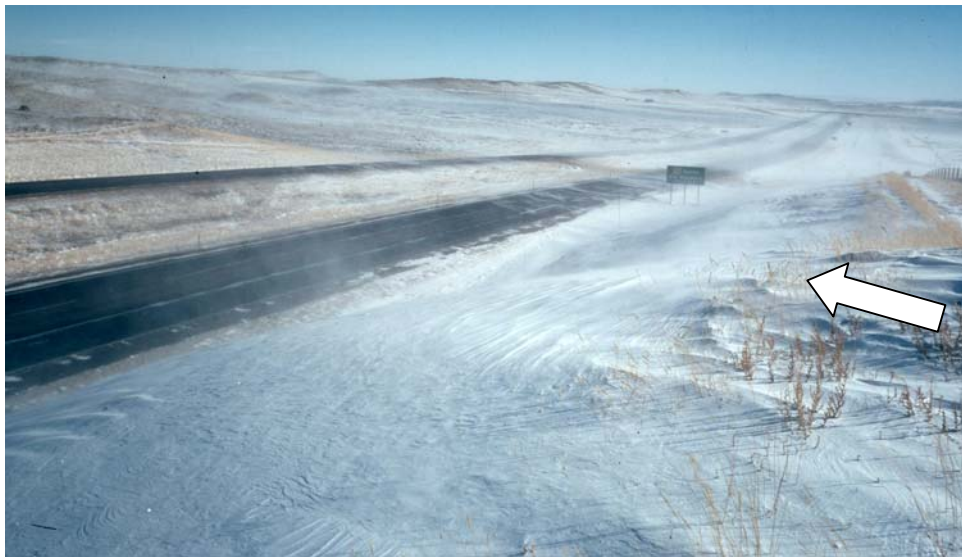
Figure 2.13. This photo taken from the center of the protected area shows the improved visibility downwind of 3.8-m (12-ft) fences, located outside of the field of view to the right (arrow indicates wind direction). The end of the fence system coincides with the abrupt change in conditions just beyond the information sign (Mile 254, Wyoming I-80). (From Tabler 1986).
