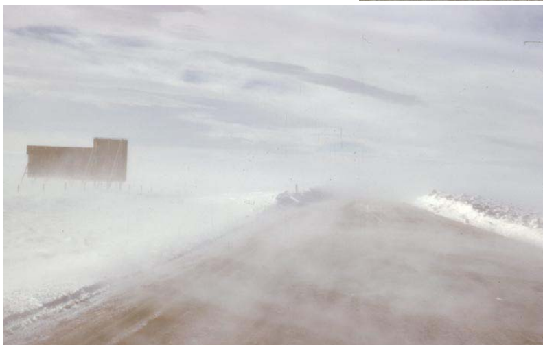
Figure 4.5. This tall billboard is causing a snowdrift on the road even though it is 30 m (100 ft) from the shoulder (Tabler 1994). Plow drivers had not realized that the sign was causing this drift.
