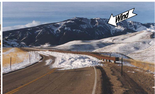
Figure 8.37. W-beam beam safety barrier causes snowdrifts and obstructs plow cast (left from Tabler 1994).
