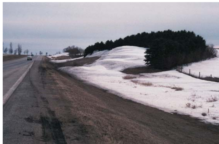
Figure 7.14. Wrapping a planting around a road cut causes large drifts on the road at the ends of the trees.
