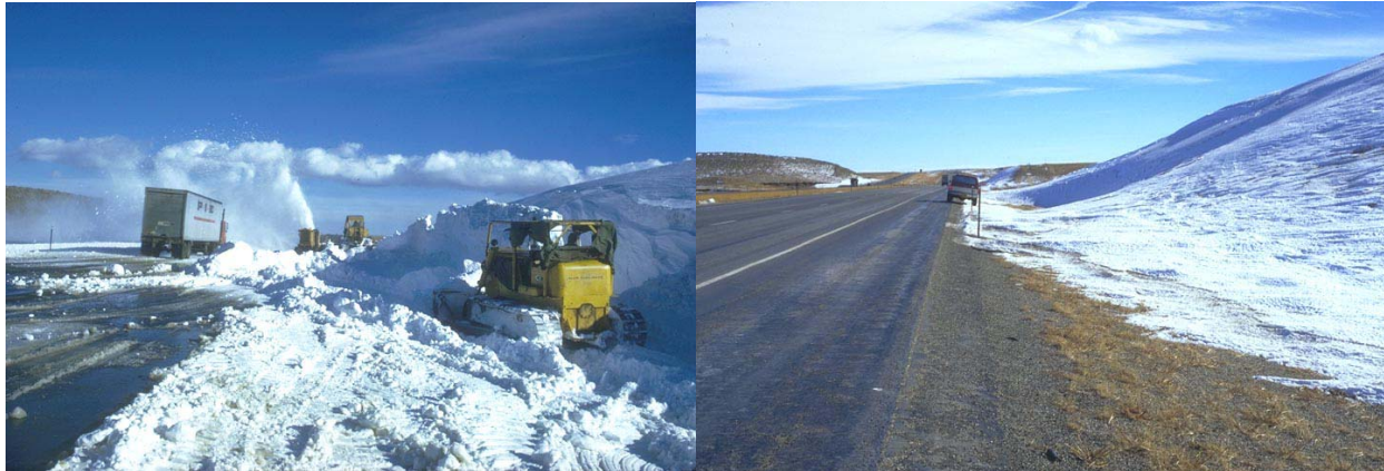
Figure 2.8. Snow accumulation at Wyoming I-80 Mile 274.9 in 1970 before fencing (above), compared with conditions typical of the 31 years since fences have been in place (upper right). At the time of the lower photo, the drift formed by the 3.8-m-tall (12.4 ft) fence at this site was 6 m (20 ft) deep and contained about 80 metric tons per meter of fence length (27 tons/ft). (From Tabler 1973a).
