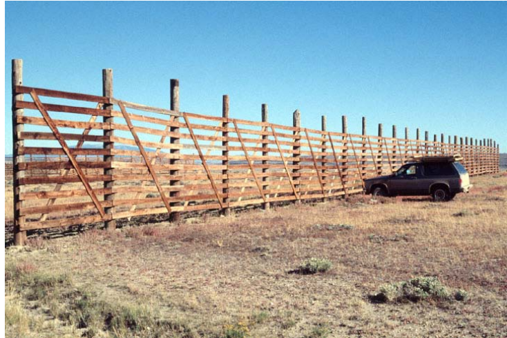
Figure 6.24. Rails supported by poles were used for this 3.3-m-tall (10-ft) fence (Tabler 1994).
