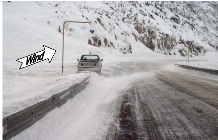
Figure 8.40. Shirttail drifts form at the ends of safety barrier.
