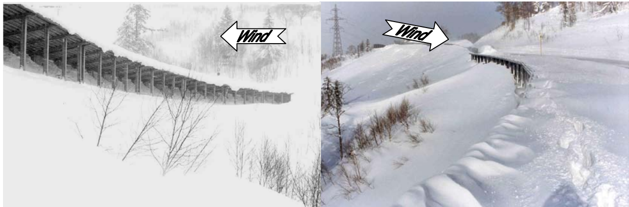
Figure 6.3. Solid barrier near Nakayama Pass, Hokkaido, Japan, causes snow to be deposited on the slope below the road, diffuses snow vertically, and retards deposition on the road (Tabler 1994). Right photo courtesy of Tetsuya Uchiya, Hokkaido Development Bureau.
