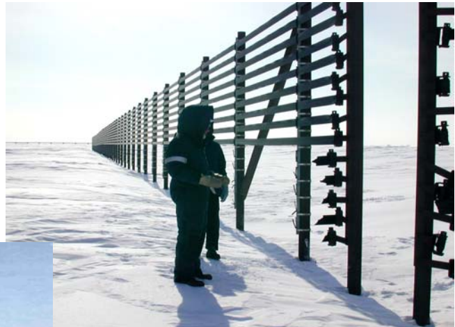
Figure 6.47. In areas with strong winds, stays or vibration dampeners should be used to limit unsupported spans to 1.5 m (5 ft).
