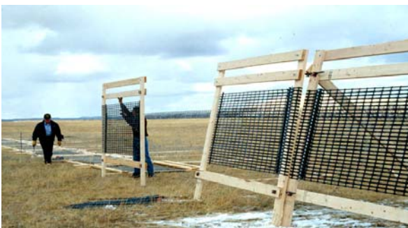
Figure 5.40. Design for seasonal fences 2.0 m (6.5 ft) and 2.4 m (8.0 ft) tall (left Tabler 1994).
