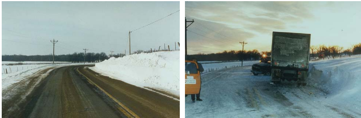
Figure 2.1. The snowdrift on this curve reduced sight distance and prevented evasive maneuvers that might have prevented this fatal crash.
