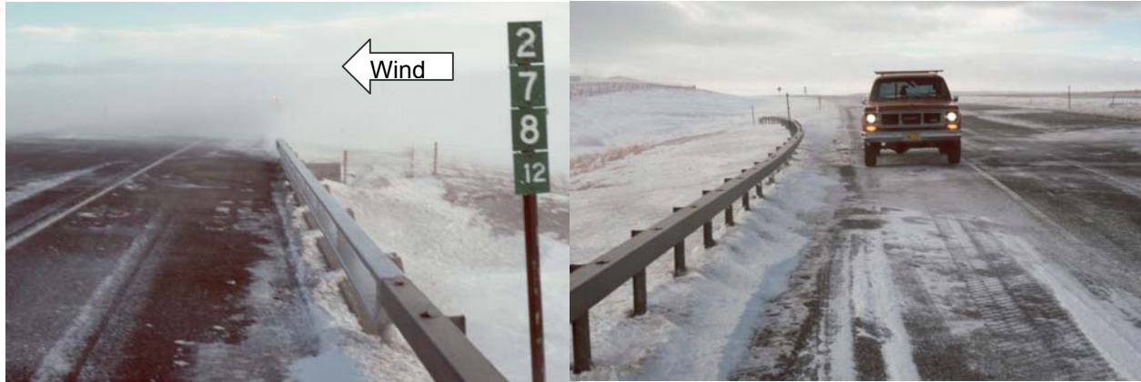
Figure 5.26. This visibility transition is at the end of a system of 3.8-m-tall (12.4-ft) snow fences on Wyoming I-80. The left view shows the abrupt change in conditions at end of the fence system coinciding with the far side of a machinery underpass. The right view shows conditions within the protected area at the same time, looking in the opposite direction. (Tabler 1994).
