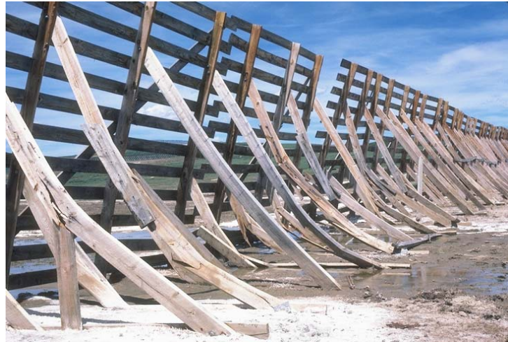
Figure 6.9. Knee braces are required to prevent long braces from being damaged by snow settlement pressure, as occurred behind this 3.6-m-tall (12-ft) fence of an earlier design.
