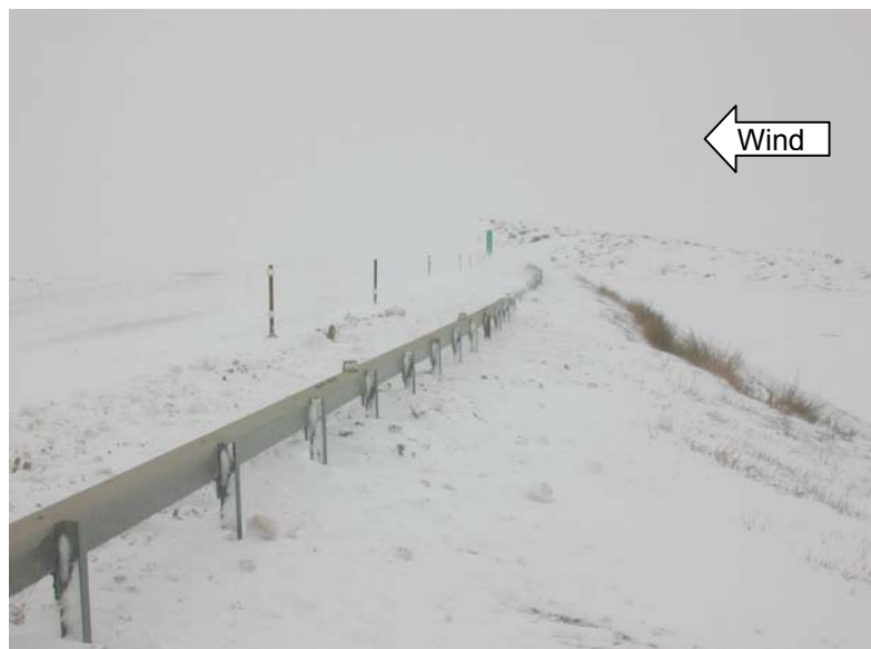
Figure 8.15. Snow depth increases with slope steepness. The effect shown here may be exacerbated by the unmowed vegetation on the steeper slope.
