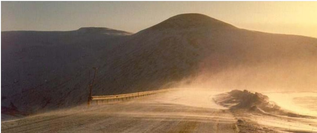
Figure 8.16. Safety barrier on embankments cause serious snow drifting problems. Photo courtesy Craig Shelton, Northern Region, Alaska Department of Transportation and Public Facilities.
