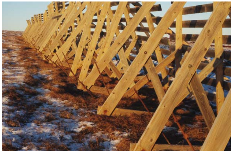
Figure 6.16. Seasonal freezing and thawing has jacked out the rebar anchoring this 4.3-m-tall (14-ft) fence near Nome, Alaska.
