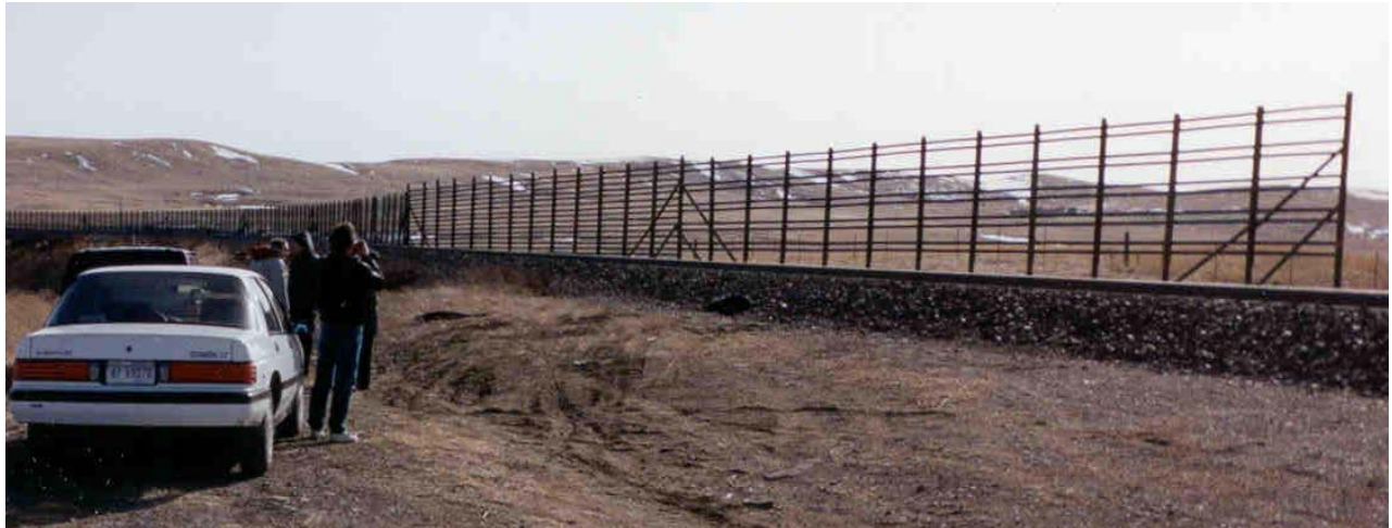
Figure 6.37. Composite polymer/wire rail was used to phase out wind protection over the last 90 m (300 ft) of this fence to prevent an abrupt transition from protected to unprotected conditions.
