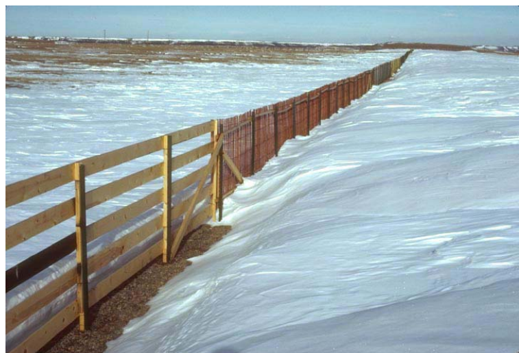
Figure 3.52. Horizontal slats reduce the tendency for snow deposition near the fence (Tabler 1986).
