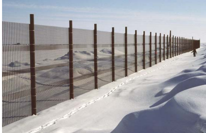
Figure 6.30. Snow fences 4.6 m (15 ft) tall at Prudhoe Bay, Alaska, utilize UX3100 high-density polyethylene snow fencing manufactured by the Tensar Corporation (Tabler 1994).
