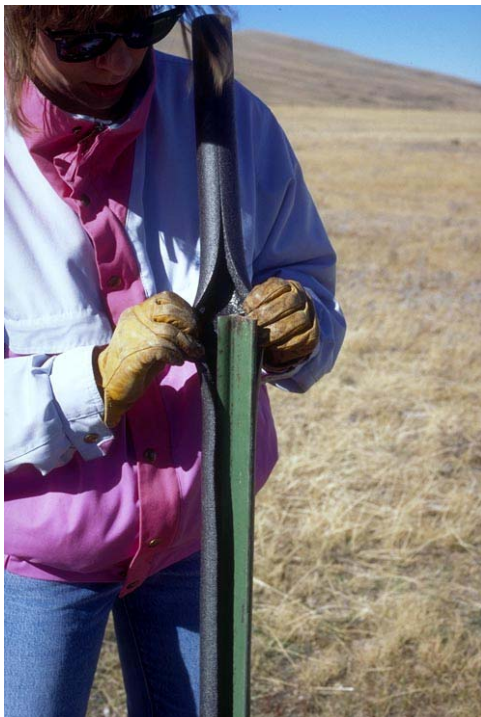
Figure 6.52. Foam pipe insulation slipped over a steel T-post provides a better grip on fencing than wooden lath (Tabler 1994).
