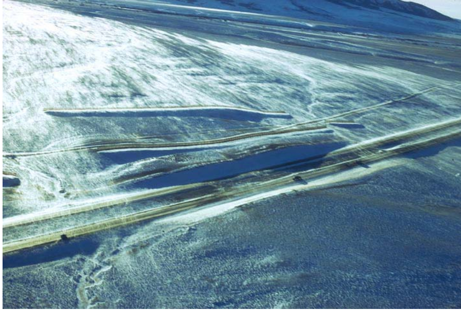
Figure 2.10. Very little blowing snow is seen escaping the two 3.8-m (12.4-ft) fences at Mile 263.0, Wyoming I-80 (Tabler 1973a). At the time of this photo, the lead fence was about 60% full. Photo by Robert L. Jairell.
