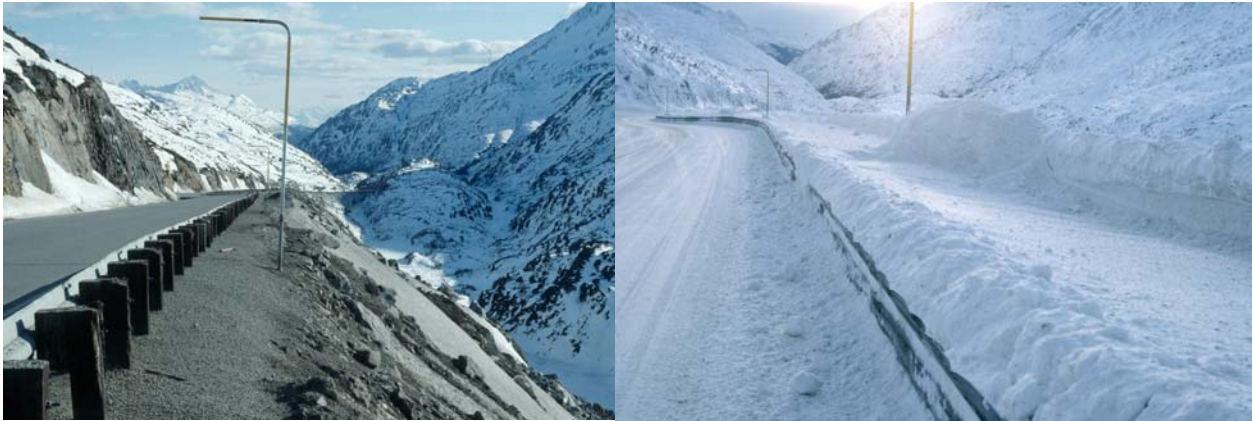
Figure 8.31. A wide bench outside of guardrail promotes snow accumulation.
