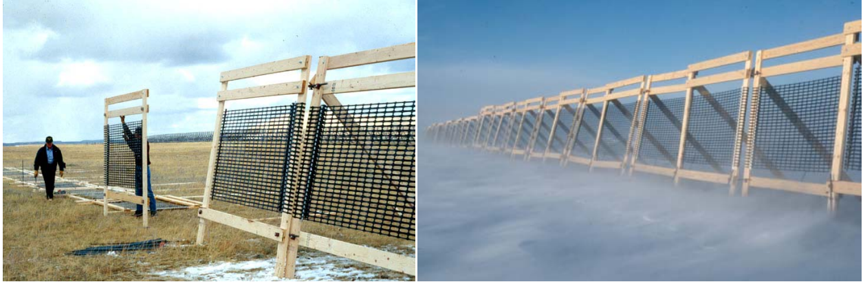
Figure 6.53. The 2.0- and 2.4-m-tall (6.5- and 8-ft) patented portable fence design uses a wooden framework to support the Tensar ® fencing material (left from Tabler 1994). The 2.4-m version is shown in these views.
