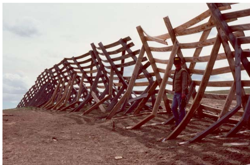
Figure 6.78. Damage to the buried fence shown in Figure 6.74 (Tabler 1986b).
