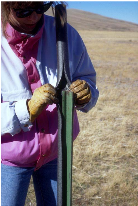
Figure 5.39. Foam pipe insulation slipped over a steel T-post provides a better grip on fencing than wooden lath (Tabler 1994).
