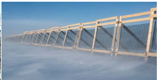
Figure 5.40. Design for seasonal fences 2.0 m (6.5 ft) and 2.4 m (8.0 ft) tall (left Tabler 1994).
