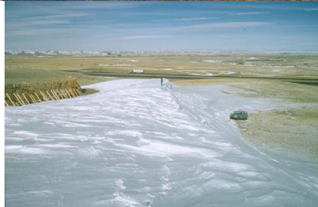
Figure 2.8. Snow accumulation at Wyoming I-80 Mile 274.9 in 1970 before fencing (above), compared with conditions typical of the 31 years since fences have been in place (upper right). At the time of the lower photo, the drift formed by the 3.8-m-tall (12.4 ft) fence at this site was 6 m (20 ft) deep and contained about 80 metric tons per meter of fence length (27 tons/ft). (From Tabler 1973a).
