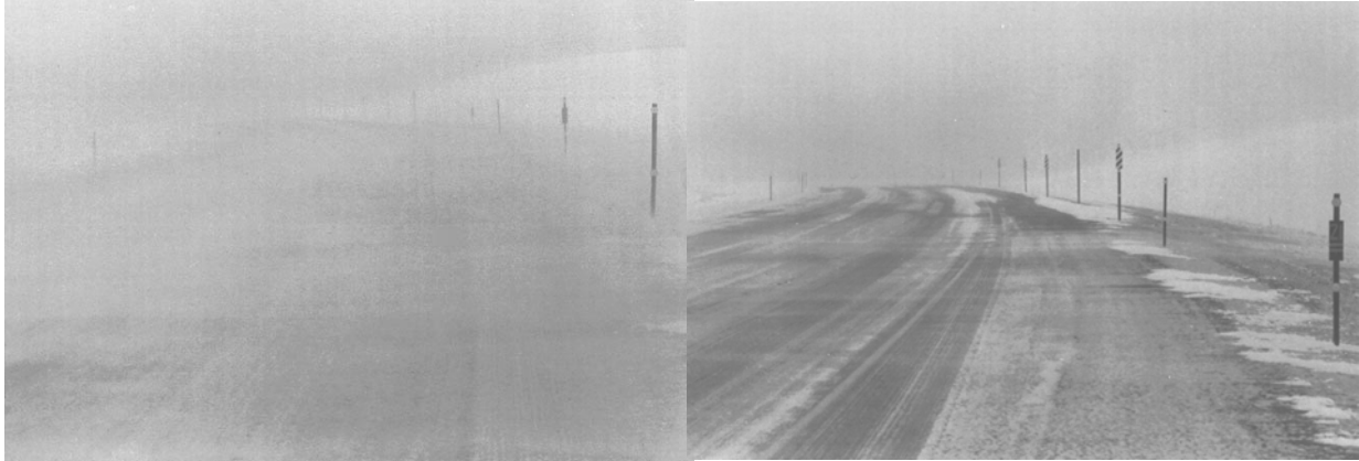
Figure 2.12. Improved visibility downwind of a 3.8-m (12.4-ft) snow fence during moderate drifting. The left photo was taken 60 m (200 ft) outside of the protected area. The right photo was taken a few minutes later, standing at the boundary of the protected area. Photos by Keith Rounds, Wyoming Department of Transportation. (From Tabler 1973a).
