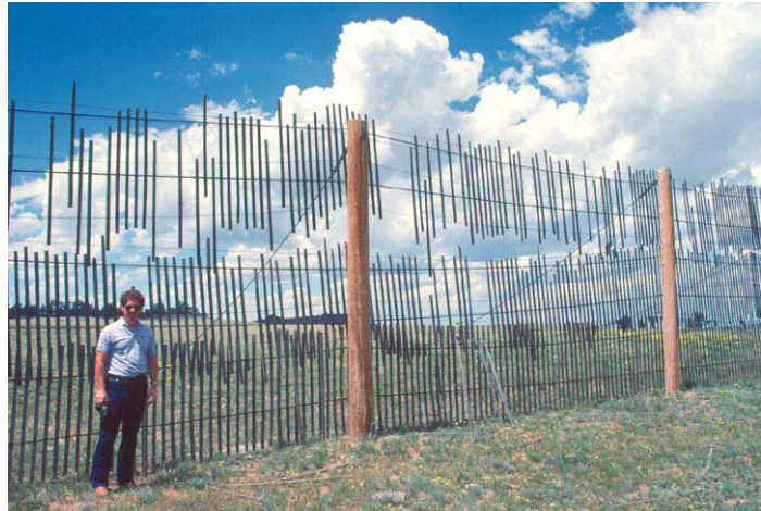
Figure 6.26. Lath fencing is unsuited for tall permanent fences because the slats fall out of the wire loops after several years of service (Tabler 1994).
