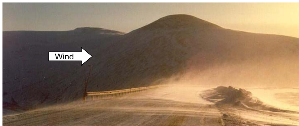
Figure 5.13. Safety barrier causes snowdrifts. Left view shows W-beam rail, right view is concrete median barrier (Tabler 1994). Arrows indicate wind direction.
