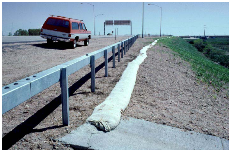
Figure 8.39. Box-beam rail with temporary curb (Tabler 1994). Temporary curbs should be used in preference to permanent curbs under rail.
