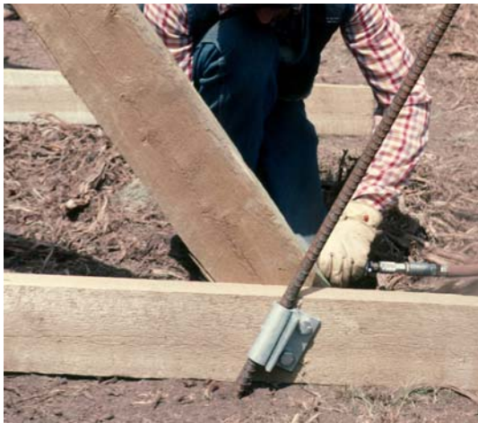
Figure 6.17. Anchor attachment for permafrost soils allows fence to move vertically in response to thawing and freezing of active layer. Dimensions are in millimeters.
