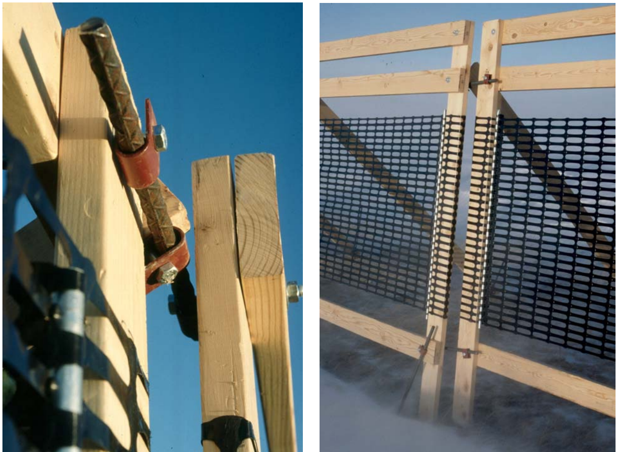
Figure 6.54. Panels are connected using the U-clips shown in Figure 6.11, with rebar pins. The 2.0-m (6.5-ft) version is shown on the left (Tabler 1994).
