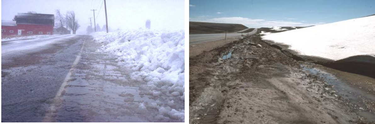
Figure 2.2. Snowdrifts can contribute to road damage by obstructing drainage and providing a source of water that can infiltrate under the pavement (left photo from Tabler 1994).
