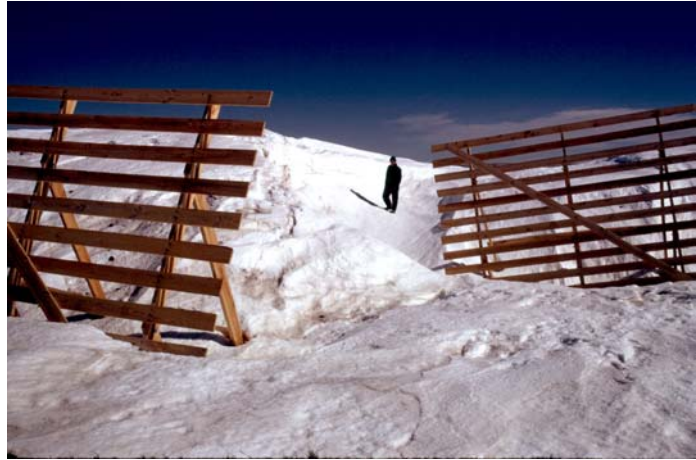
Figure 6.84. Opening in fence similar to Type A in Figure 6.83. Fence height is 3.8 m (12.4 ft)
