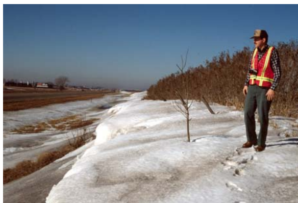
Figure 7.9. Shrubs planted at the top of a cut can be used in place of taller barriers placed farther upwind. Snow transport must be accurately determined, however, if the risk of drift encroachment is to be acceptable. (Drawing from Tabler 1994).
