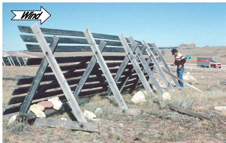
Figure 6.20. A Swedish (or Norwegian) snow fence. This 2-m (6.5-ft)-tall fence was about 45 years old at the time this picture was taken (Tabler 1986b).
