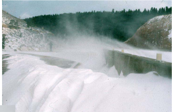
Figure 8.35. Snow blowing over the top of concrete barrier can impair motorist visibility (Tabler and Jairell 1980).
