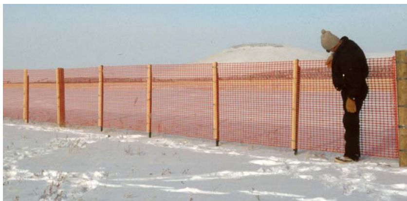
Figure 6.29. Punched and drawn high-density polyethylene "All Purpose Fence" manufactured by Conwed Plastics, Inc. (Tabler 1994).
