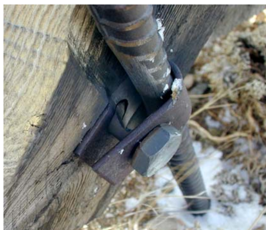
Figure 6.12. It is imperative to tighten the U-clip to prevent slippage. Right view shows rebar that has nearly rasped entirely through bolt and U-clip.
