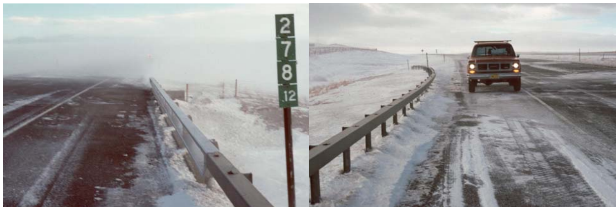
Figure 6.86. This visibility transition is at the end of a system of 3-8-m-tall (12.4 ft) snow fences on Wyoming I-80. The left view shows the abrupt change in conditions at end of the fence system coinciding with the far side of a machinery underpass. Faintly visible amber lights mark a working accident. The right view shows conditions within the protected area at the same time, looking in the opposite direction.
