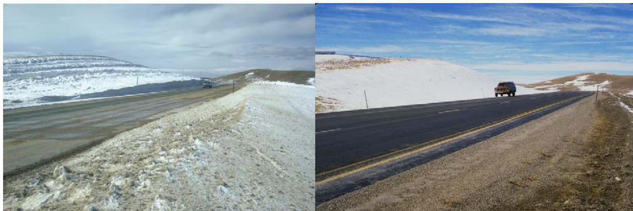
Figure 2.9. Snow accumulation at Wyoming I-80 Mile 269.5 in 1970 before fencing (upper left), compared with conditions typical of the 31 years since fences have been installed (right). The lower view shows a 3.8-m (12.4-ft) Wyoming fence with snow accumulation on the same date at another location. (From Tabler 1973a).
