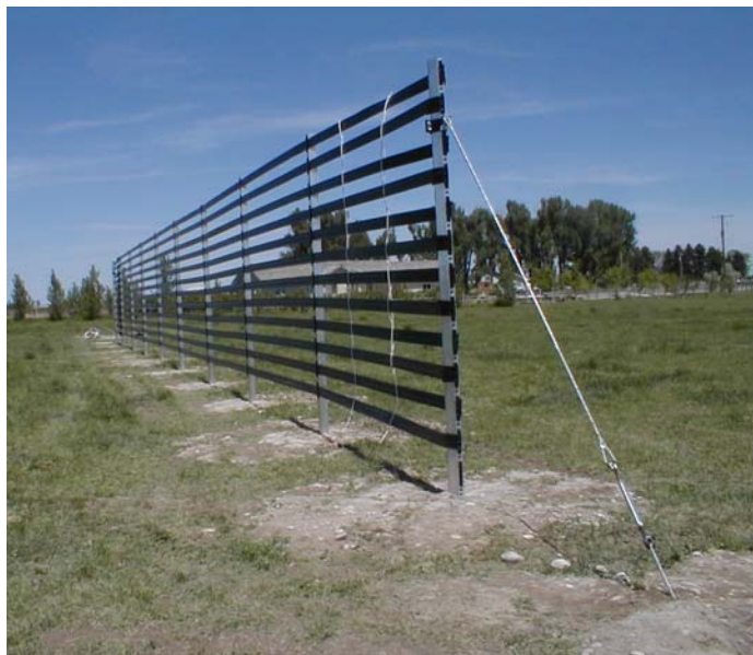
Figure 6.44. Perma-Rail® slotted aluminum post and bracket system. Note use of guys in place of braces. Photos courtesy of Perma-Rail International.
