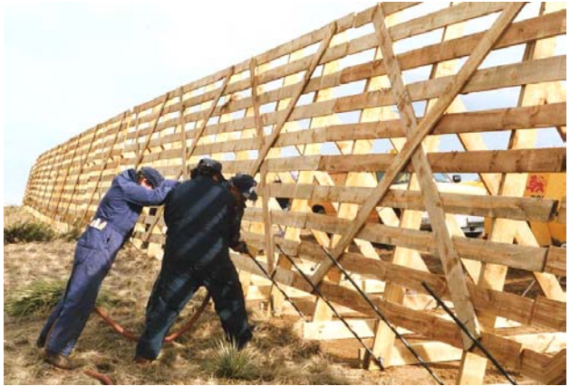
Figure 5.28. 3.0-m (10-ft) Wyoming snow fence.
