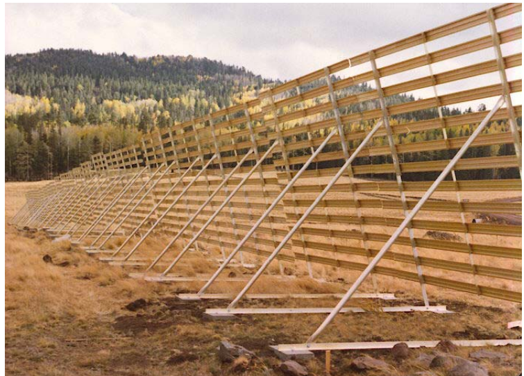
Figure 6.7. Aluminum Wyoming-type snow fence developed by the Arizona Department of Transportation. Photo courtesy Arizona Department of Transportation.
