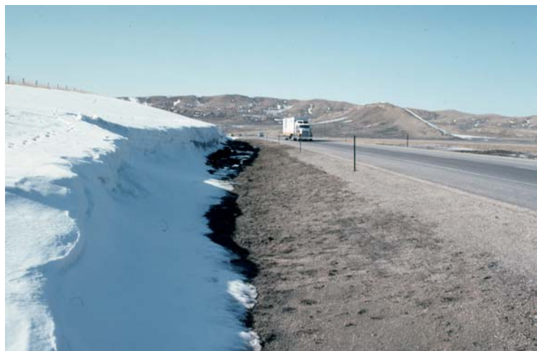
Figure 8.23. Guidelines recommended in Figure 8.22 maximize snow storage in cut and reduce possibility that drift will encroach on roadway.
