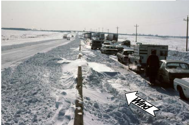
Figure 8.36. Snowdrift caused by concrete barrier blocked Interstate Highway 25 in Colorado, during the Christmas Blizzard of 1982 (Tabler 1994).
