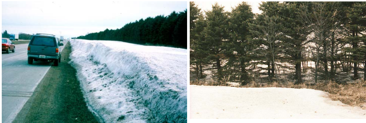
Figure 7.15. Deep drift on road resulted from needle loss of mature spruce trees planted 30 m (100 ft) from road edge.
