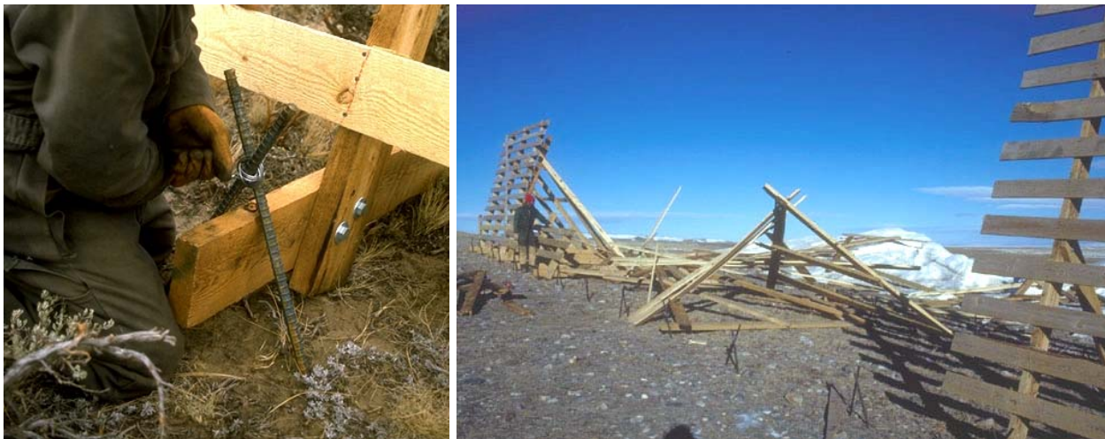
Figure 6.14. Crossed and wired rebar should not be used to anchor Wyoming fences (Tabler 1994).
