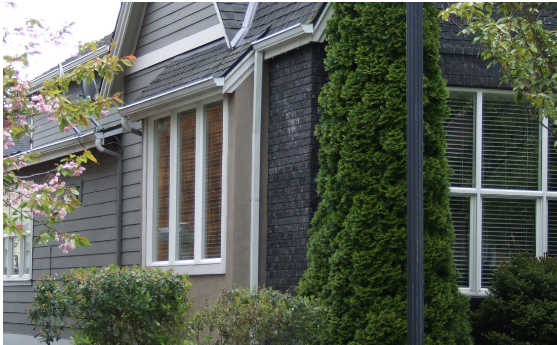
MA-2 Brick finish terminates at inside corner of window bay.
