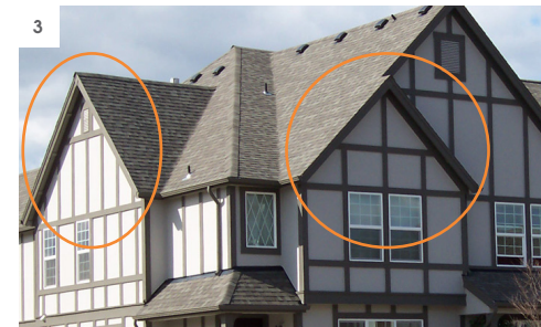
(1) The bulk of the roof is reduced by the use of multiple dormers which provide a rhythm and align with the space between the columns below. (2) The low slope of these secondary roof forms reduce the perceived scale of this large dwelling. (3) Secondary roof forms at corner lots present two frontages to the street. The sub-gables, shown here, moderate the scale of the primary roof and increase compatibility with neighboring houses.
