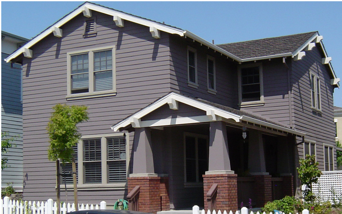
RF-3 Roof of porch matches style and pitch of primary roof.
