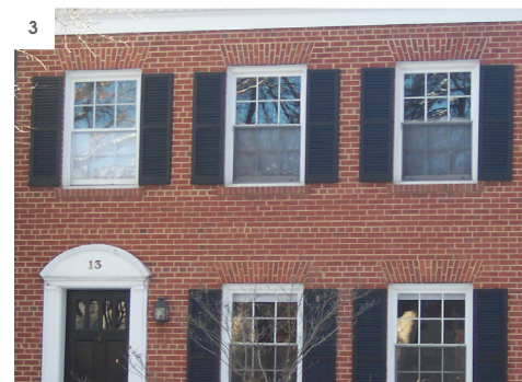
(1) Contrasting paint color of trim highlights this window. (2) Minimal flashing detail at window head is appropriate to this contemporary design. (3) Shutters and door surround are all appropriate trim features to the style of this dwelling.
