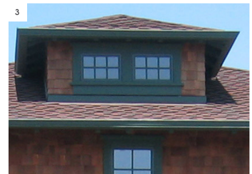
(1) Projecting front room at ground floor follows roof line and pitch of primary structure. (2) Large street-facing shed dormer brings light to this second floor which has been built into the primary gable roof. (3) Roof of dormer matches style and pitch of primary roof, creating design harmony within the structure.
