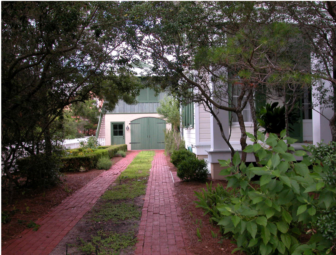
AS-3 This driveway is finished in brick pavers which functions both as a surface to park cars and as a pathway between the accessory garage structure and the house.
