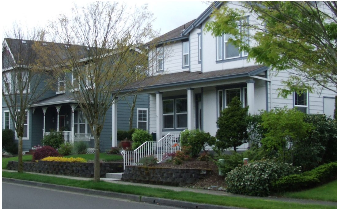
LF-1 A combination of retaining walls and tiered landscaping stabilize the slope of this front yard.
