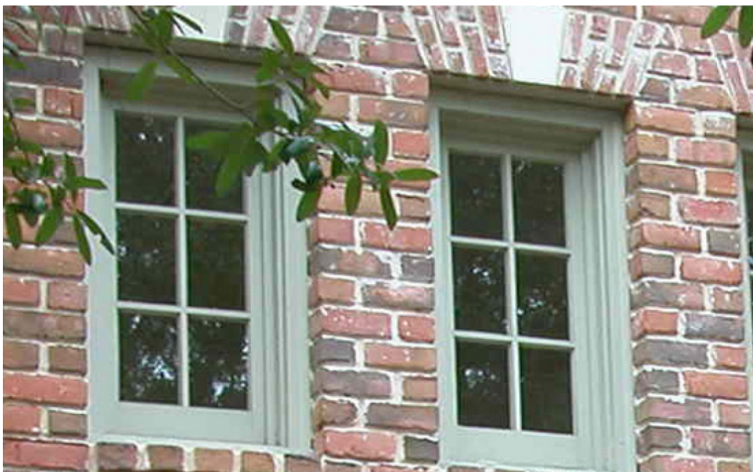
OP-6 These windows, set back in the wall, articulate the depth of the masonry, adding a level of detail.
