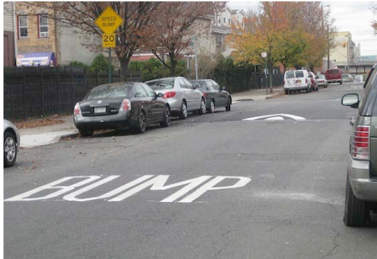
Signs and pavement markings should be used to warn approaching vehicles of upcoming speed humps. (streetsblog)
