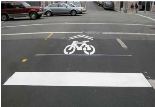
A defacto bike box is created by moving the stop bar 10’ back from the crosswalk at signalized intersections. (StreetsblogSF)
