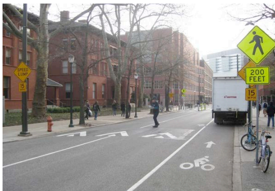
Speed humps are used on 34th Street south of Walnut Street to slow approaching vehicles before a midblock pedestrian crossing.
