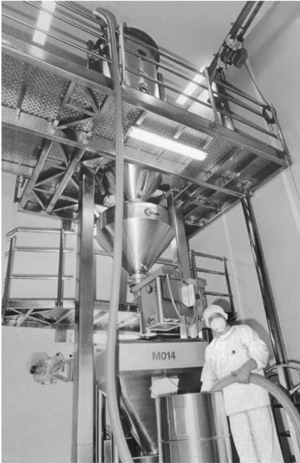
Figure 43 Integrated system. (Courtesy of the Glatt Group.)
