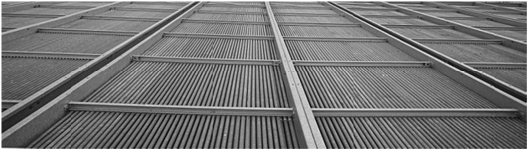
FIGURE 1.12 Air-cooled condenser. (Courtesy of GEA Iberica S.A., Vizcaya, Spain.)
