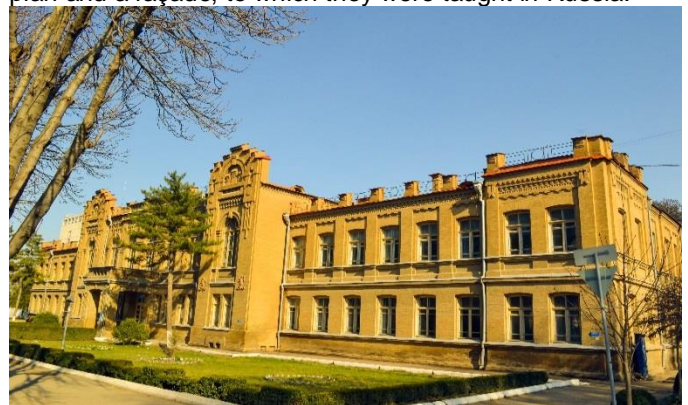
Fig. 1. Building of Girl's school in Samarkand.
