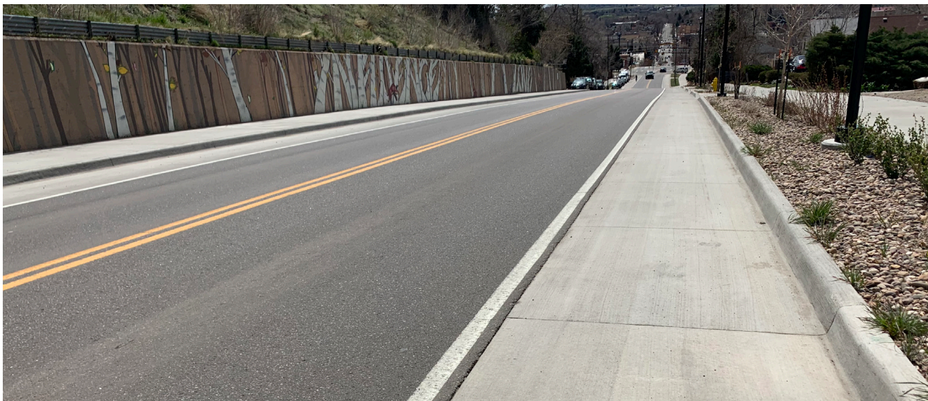
Figure 2-1: Gutter Extended Full Width of Bike Lane in Golden, CO
