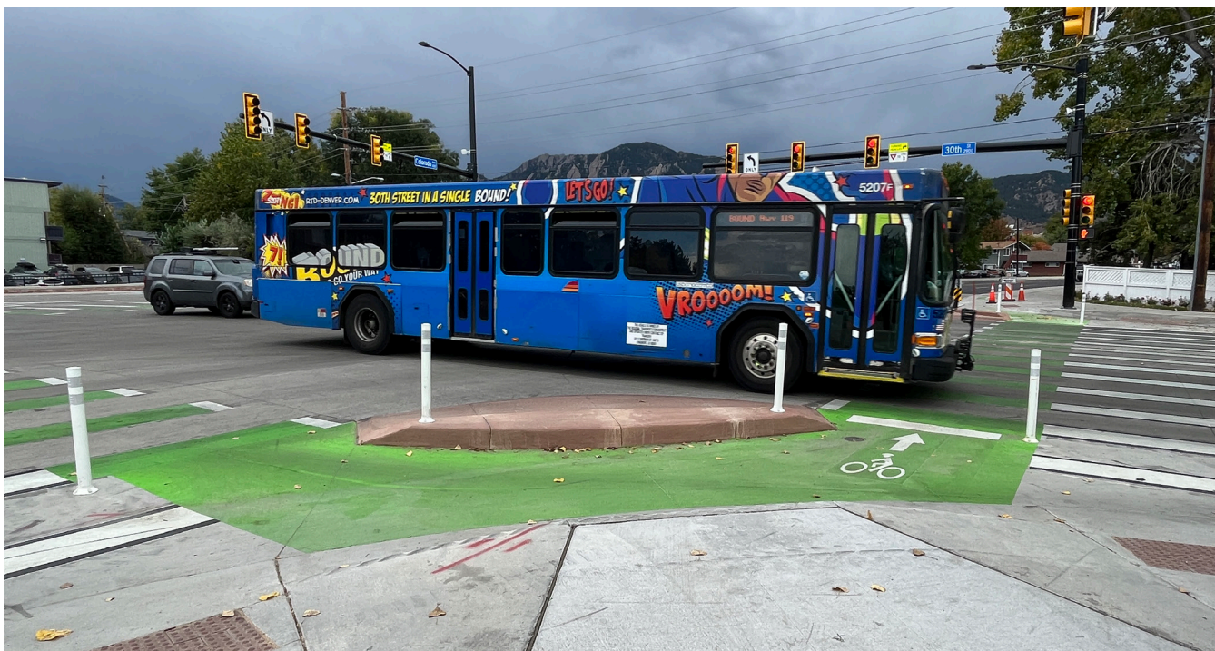
Figure 3-11: Protected Intersection in Boulder, CO
