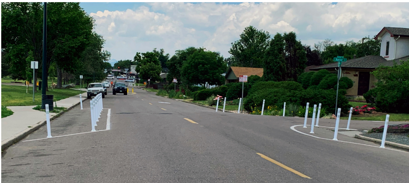
Figure 4-1: Curb Extensions on Byron Pl in Denver
