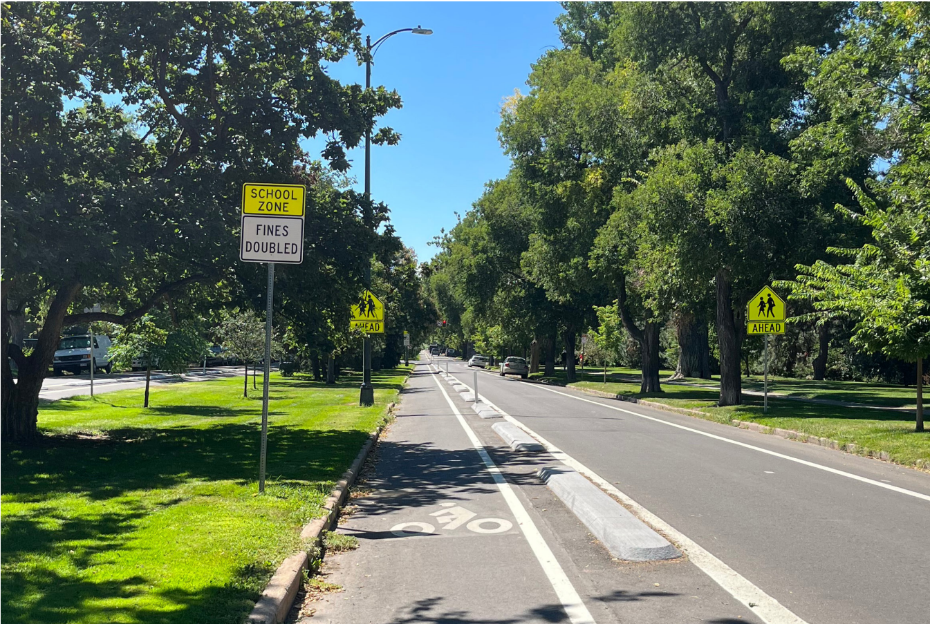
Figure 3-5: Protected Bike Lane with Standard Sign Placement
