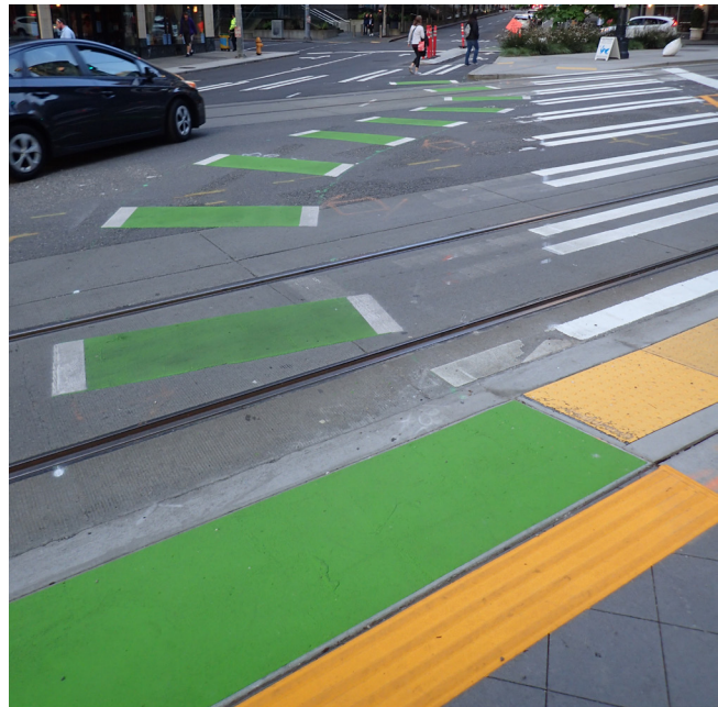
Figure 5-3: Bicycle Facility Crossing Rail Line in Seattle, WA
