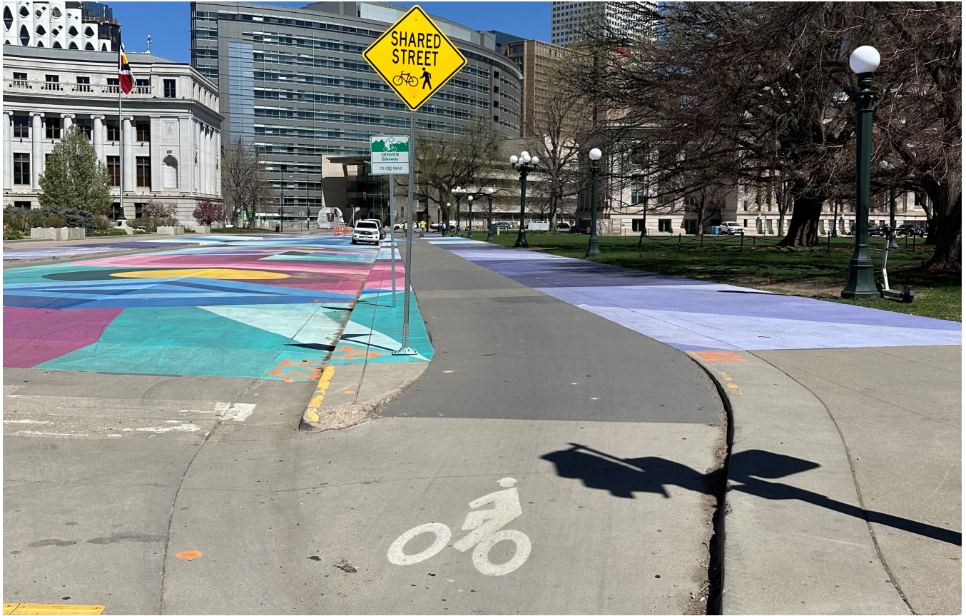
Figure 5-4: Transition from Conventional to Sidewalk-Level Bike Lane
