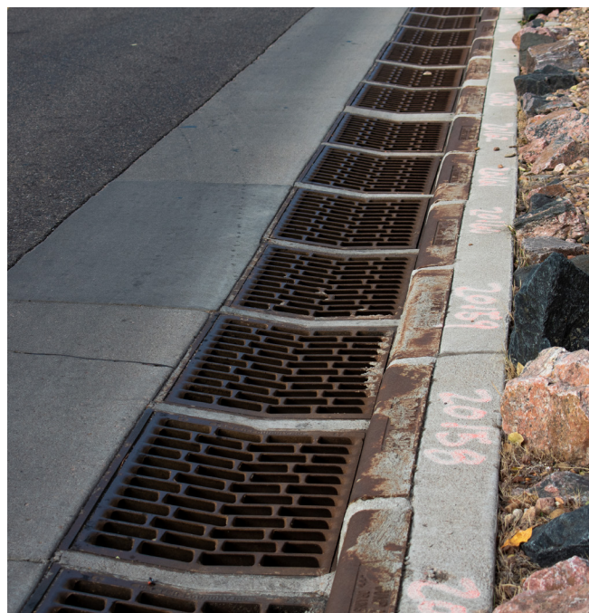
Figure 2-3: Bicycle-Friendly Inlet Grates
