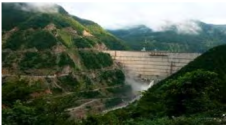
Plate 11.2. Inguri Dam in Georgia. Image sourced from [12].
