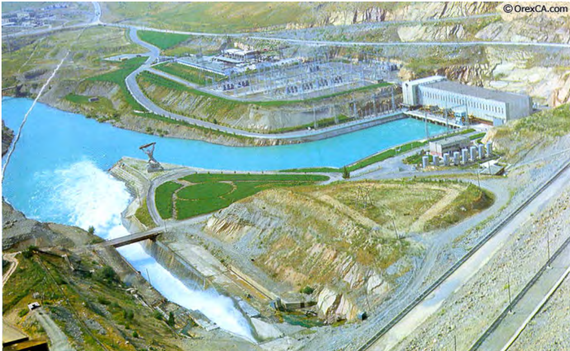
Plate 11.1. Charvak hydroelectric facility in Uzbekistan. Illustration from [11]. Reproduced with permission.
