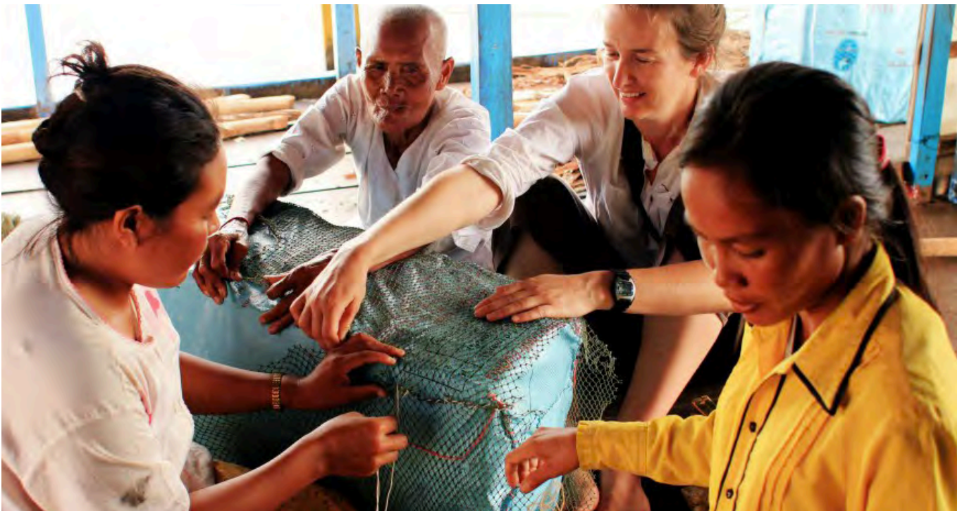
Once packed, the bags are sewn together and wrapped in damaged fishing nets to keep the bottle-bricks firmly together.
