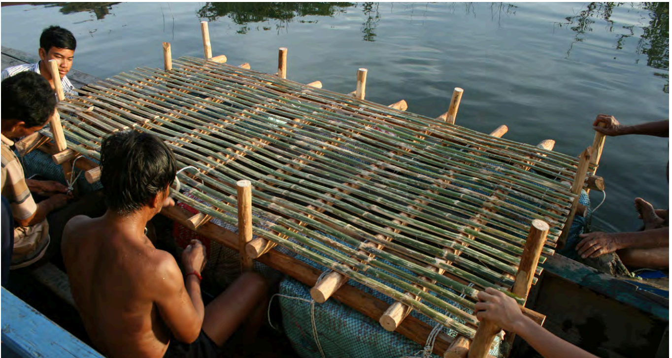
A raft is made using timber and split bamboo. The bottle-bricks are lashed underneath using rope.
