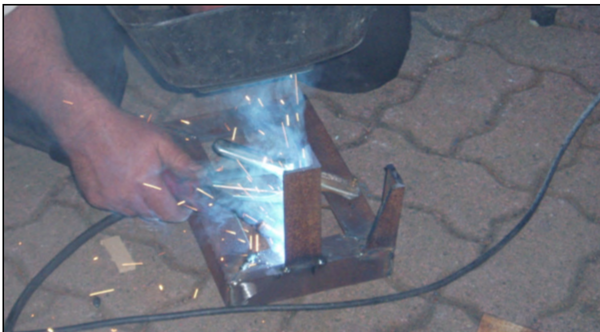
(“Angle Iron” being used to fabricate battery mounts)
