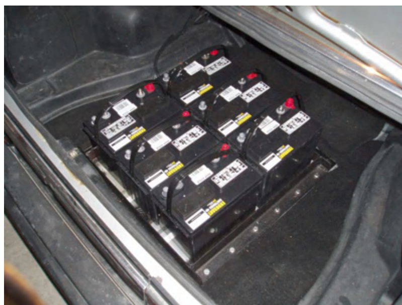
(Batteries installed in the back)
