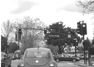
Fig. 8.1 The support arm for this traffic light is being bent by its own weight and the weight of the two traffic lights.
