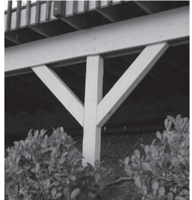
(b) Deck support in compression with a point force applied in the middle.
