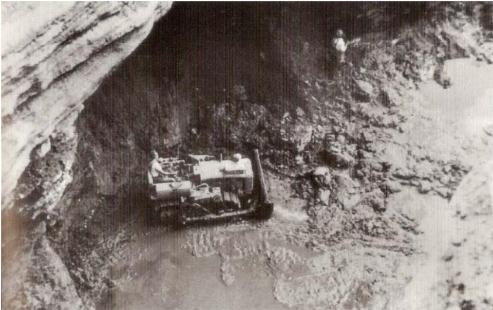
Fig 13: Bulldozers were used to fill the caverns by pushing concrete, rock, and dirt into them (Source: Applegate)
