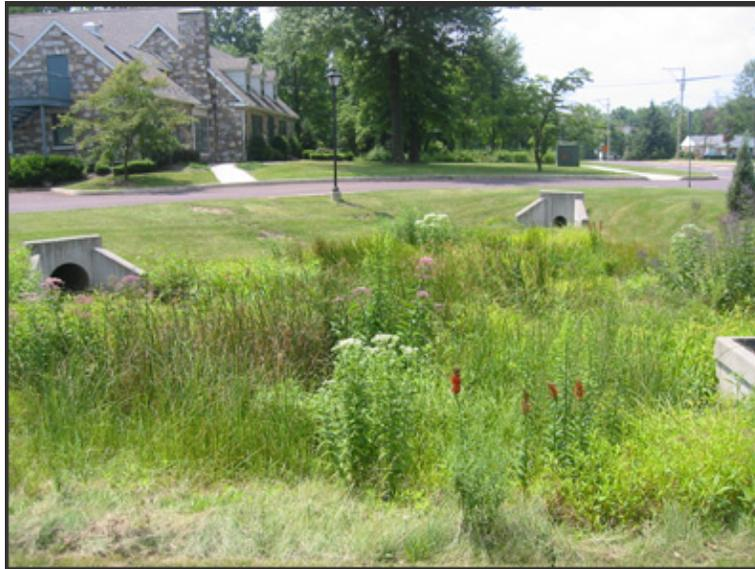
**Figure 15: Stormwater wetland.**
