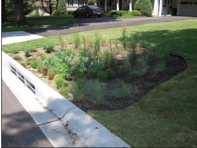
**Figure 16: Bioretention cell inlet.**
