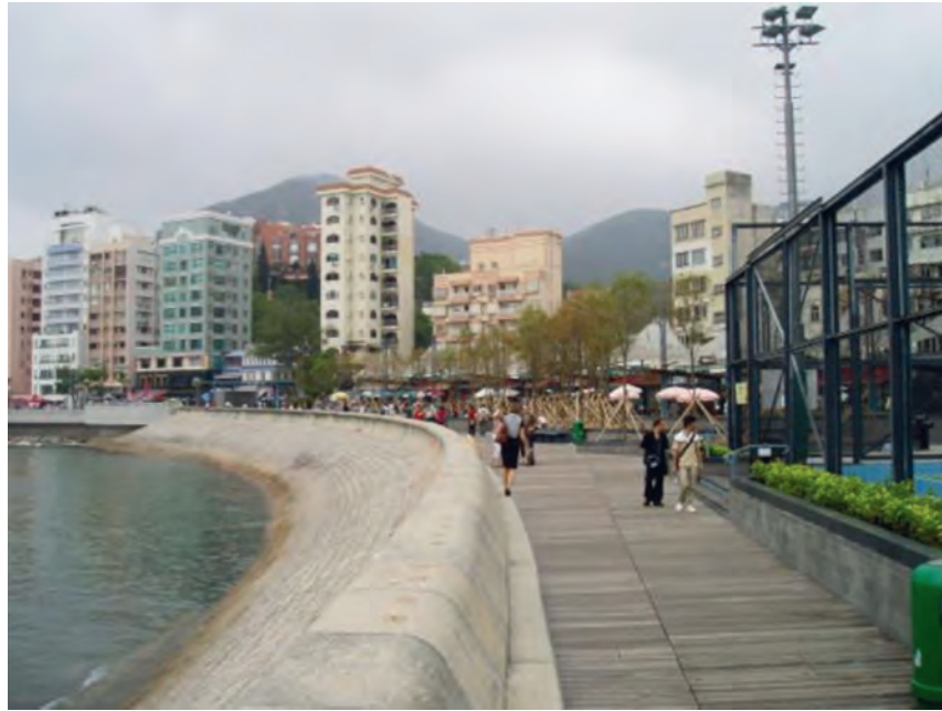
Figure 21. Seawall with wave deflector (Hong Kong).
