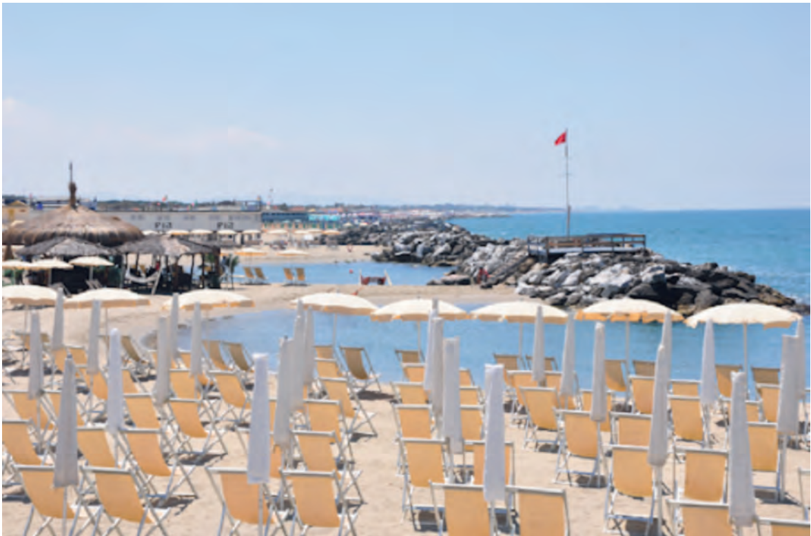
Figure 28. A series of emerged breakwaters at Marina di Pisa, Italy demonstrating poor visual impact and tombolo formation.
