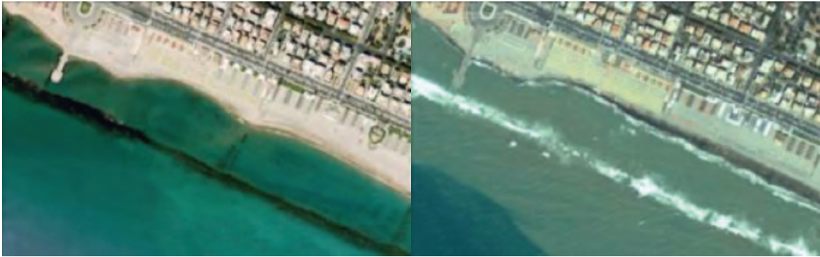
Figure 43. Artificial reef or submerged breakwater in Lido di Ostia, Rome, Italy. The 2,800 m long submerged structure was built shore-parallel in combination with submerged groynes. On the left during calm conditions, on the right with wave breaking on the crest of the structure. (SOURCE: GOOGLE EARTH)
