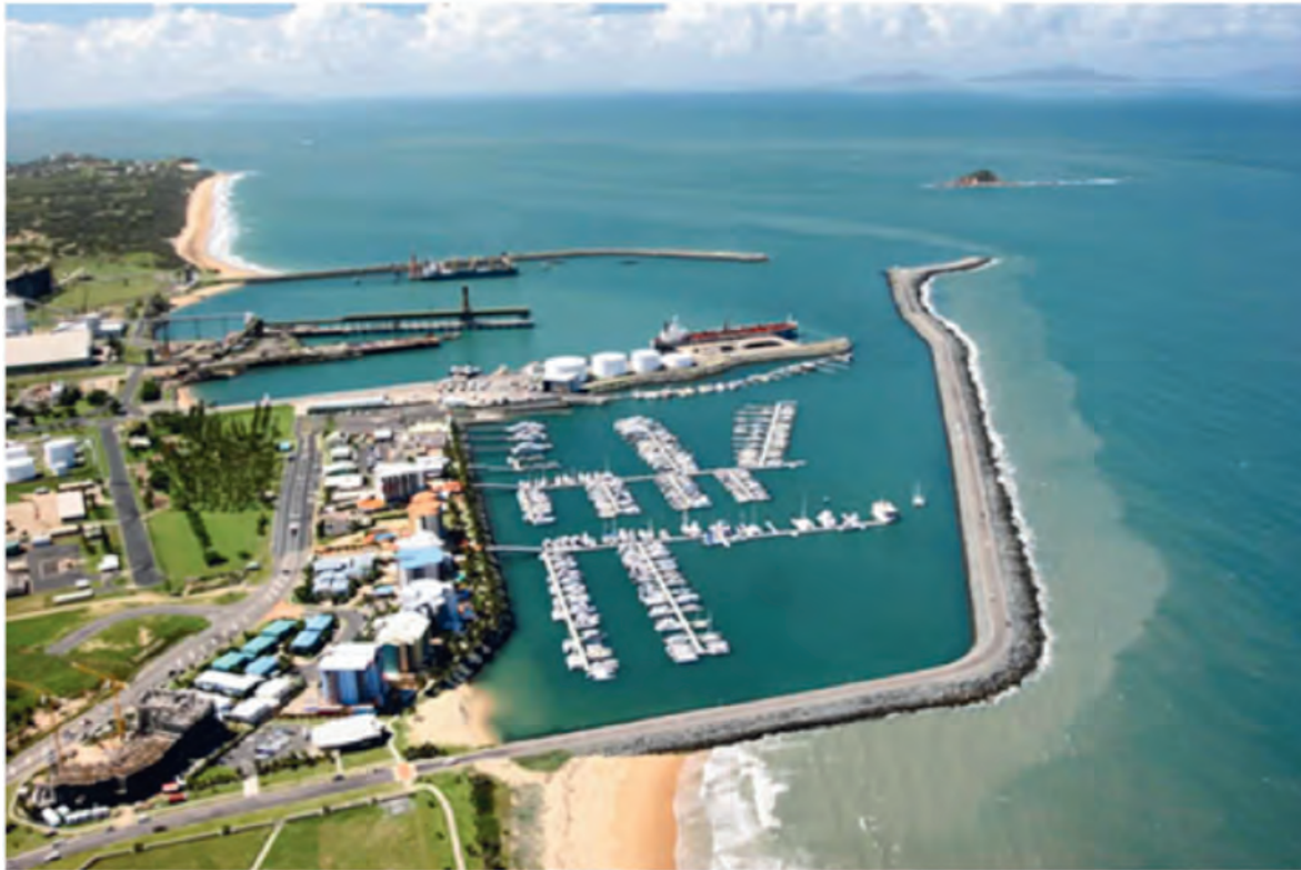
Figure 23. Breakwater at Mackay Harbour, Queensland.
