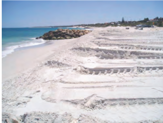
Figure 16. Beach nourishment placed to avoid dangerous erosion scarps.
