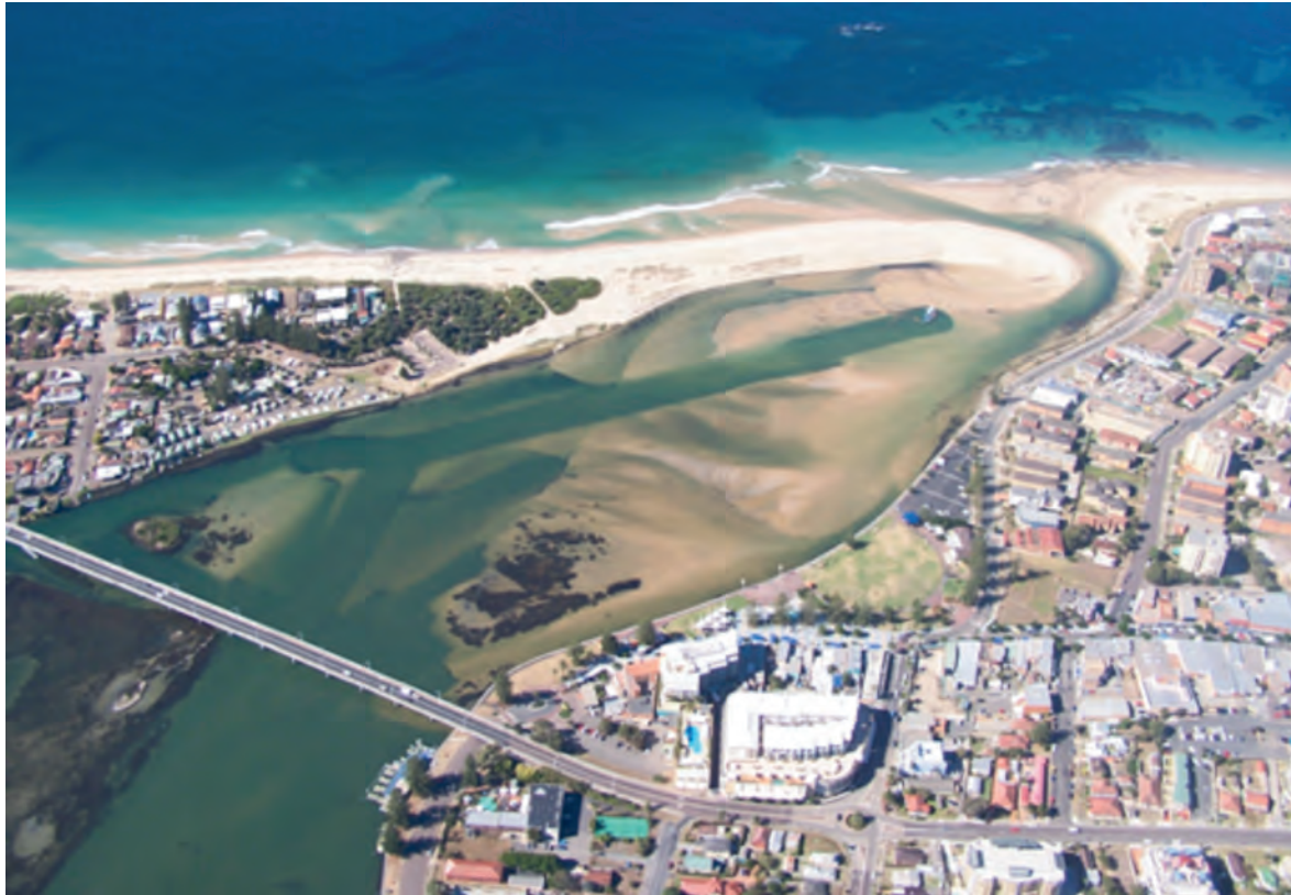
Figure 39. Council's dredger operating at The Entrance, Wyong Shire, NSW.
