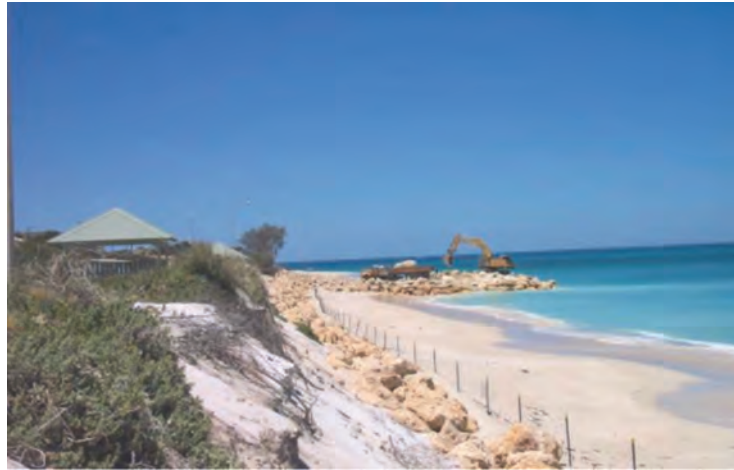
Figure 17. Rock Groyne construction at Quinns, WA.
