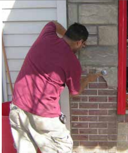
Repair deteriorated primary building materials.
