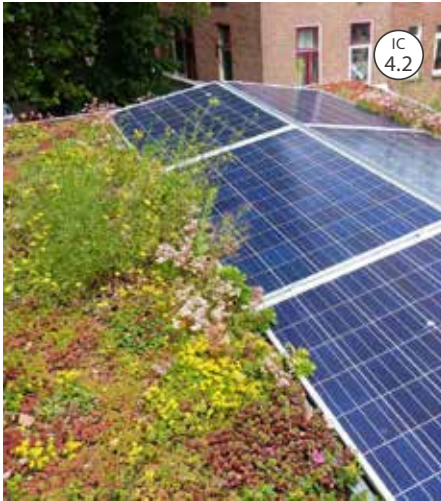
Potential for green roofs and solar panels
