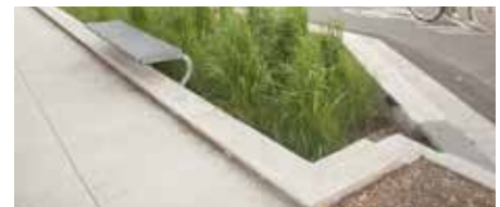
Bioretention areas are planted areas with subsurface materials that store and filter stormwater while supporting vegetation
