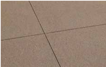
Integrally colored concrete with sandblasted finish and sawn joints can accent key features.
