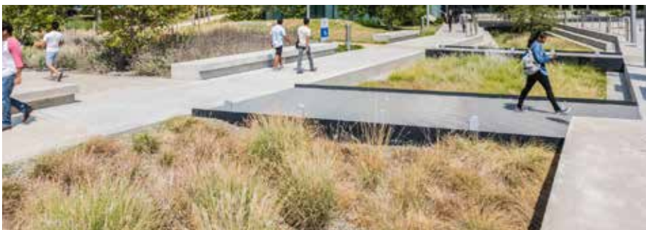
Stormwater infiltration basins should be integrated throughout the design to reduce off-site detention needs and improve water quality.
