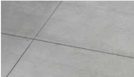
Natural colored concrete with sawn joints is a simple low-cost solution for low-use areas.
