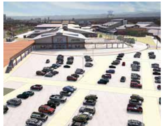
When the National Western Stock Show is not occupying this area, it will become a multi use space for events and parking.
