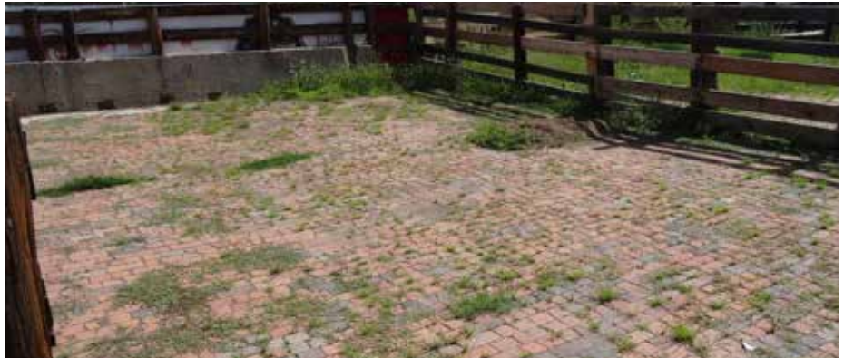
On site reused unit pavers could be utilized in pedestrian only zones near preserved structures to maintain the historic character of the Campus.
