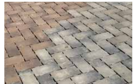
Permeable concrete unit pavers could be used where animals are prohibited to provide added stormwater infiltration.
