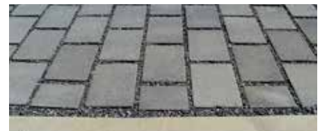
Permeable paving systems allow water to pass around pavers and infiltrate into the soil
