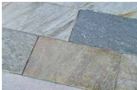
Utilized in very select pedestrian-only zones, natural cut stone provides a high level of finish and natural character.
