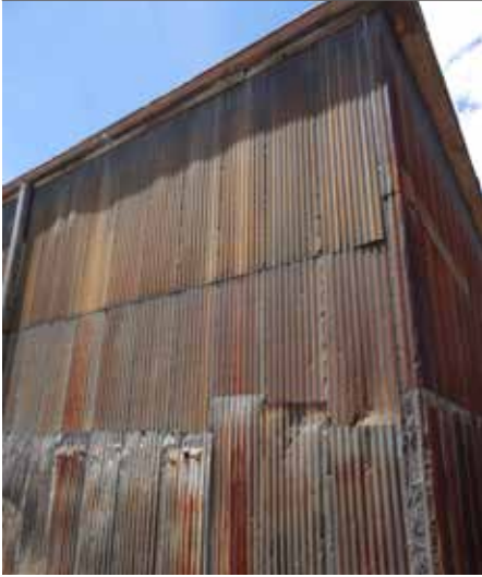
Preserve original building materials, where feasible.
