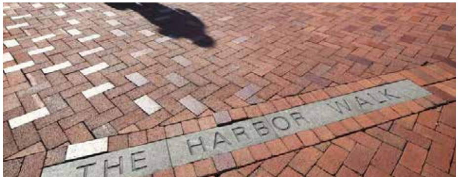
New concrete or clay unit pavers could be integrated with concrete inlays at key thresholds as a secondary wayfinding element.
