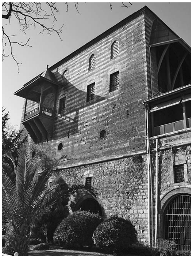
The palace of Ibrahim Pasha, the favorite grand vizier of Süleyman I, occupied a prime location on the Hippodrome of Istanbul. The Hippodrome was the main ceremonial space of the Ottoman capital, situated proximate to the Aya Sofya and the Topkapı Palace. The palace’s prime location signaled the importance and influence of Ibrahim Pasha. (Photo by Gábor Ágoston)
