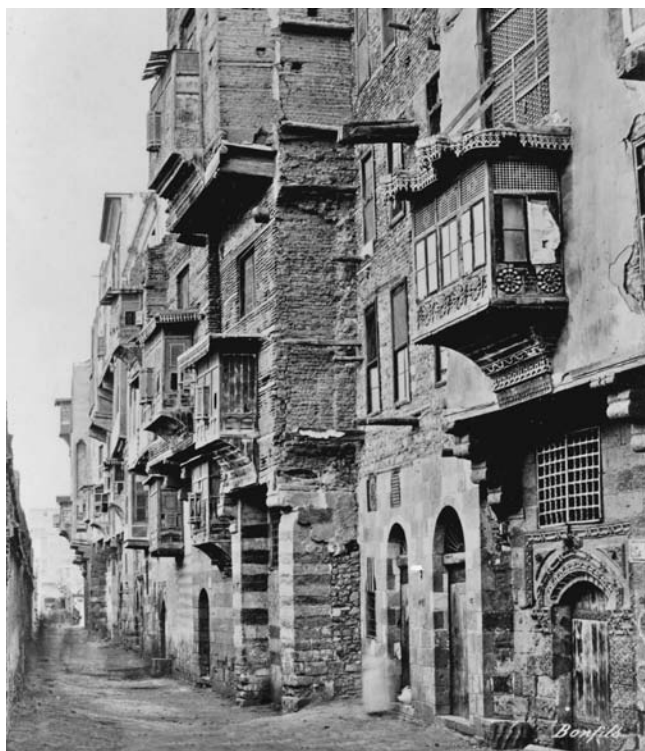
Taken in the 1880s, this photo shows a street in the Ibn Tulun quarter of Cairo. Traditionally, the houses in Cairo were several stories high and were made of mud brick with stone facades on the ground floor. The wooden window projections on the upper floors, known as mashrabiyya , allowed the women of the house to watch the street action without being seen. (Photograph by Maison Bonfils, courtesy of the University of Pennsylvania Museum, Philadelphia)
