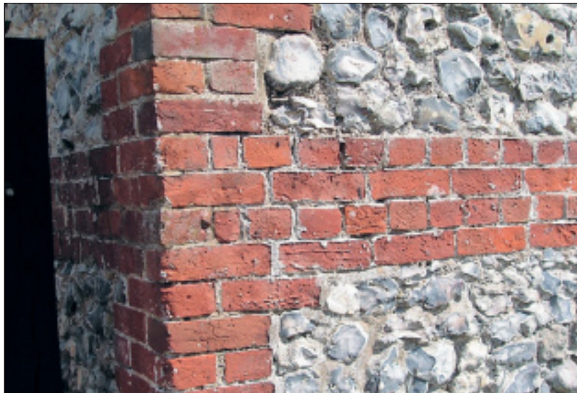
Right: Flint walling with brick quoins
