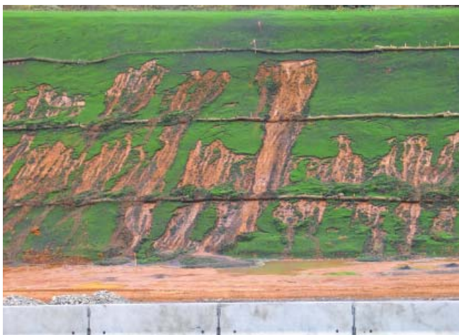
Figure 5 ~ Past approaches to revegetation often failed if the focus was on quick cover, not long-term goals. Integration of revegetation techniques into road planning and implementation increases chances of success.
