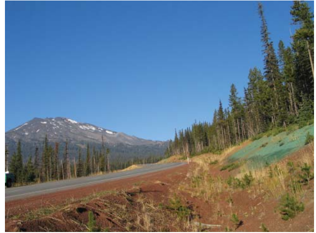
Figure 17 ~ Beginning revegetation with native species on scenic highway to Mt. Bachelor, Oregon.
