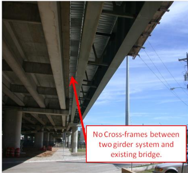
a) Twin Girder Widening
