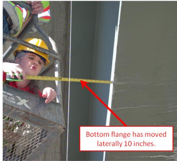
b) System Buckling
