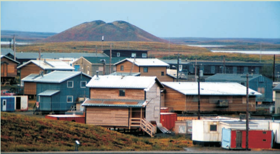
Plate 11.2 Pingo beside Tuktoyaktuk, an Inuit village on the Mackenzie Delta on the Arctic coast of Northwest Territories, Canada. The houses all stand on piles bored into the permafrost. (Photograph by Tony Waltham Geophotos)
