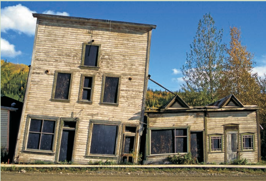
Plate 11.12 Subsidence due to thawing of permafrost, Dawson, Klondike, Alaska, USA. (Photograph by Tony Waltham Geophotos)
