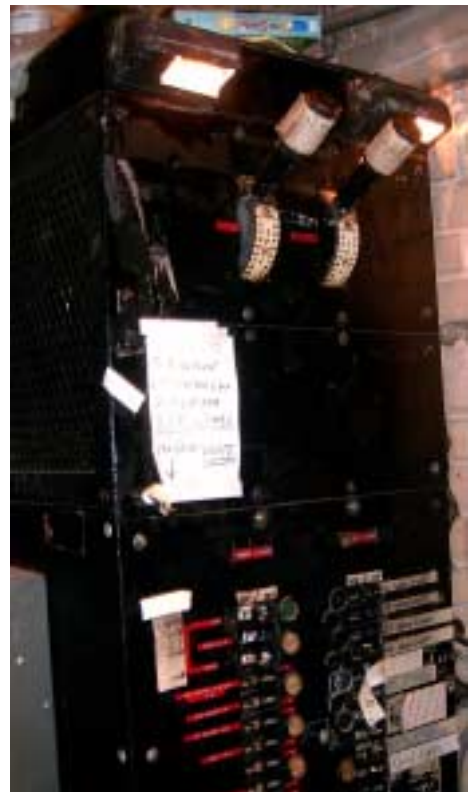
Shubert Theatre's House Light Autotransformer Board
