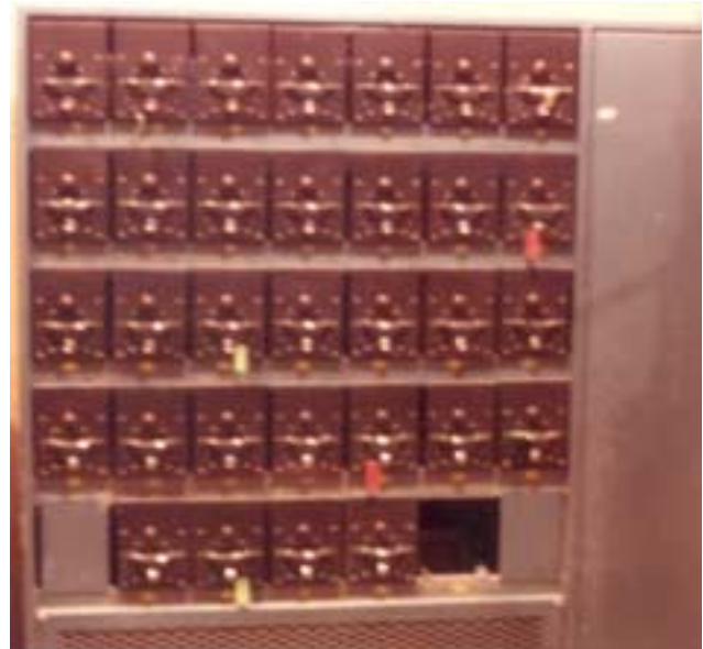
Major Controls installed dimmer Rack
