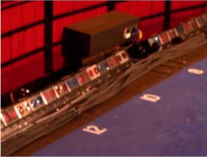
Mini Strips used as down stage footlights
