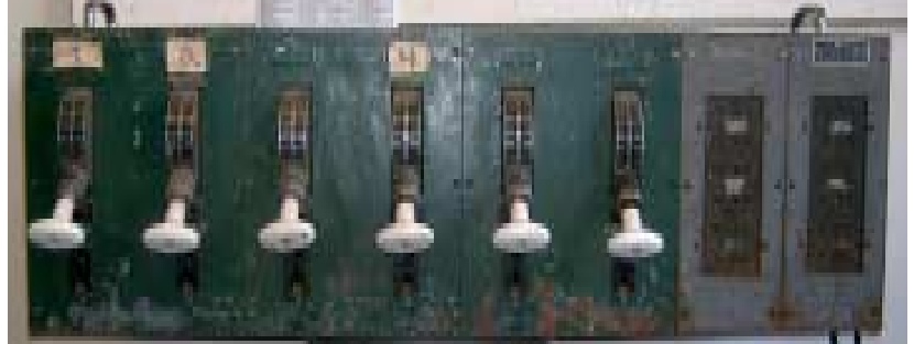
Ward Leonard “6 Pack Coffin” with stage pin load patch
