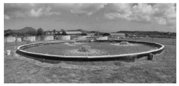
Figure 2. View of rearing tank with three vertical lift aerators.
