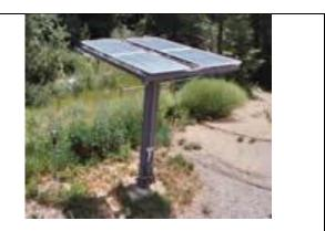
**Tracking solar panel mounts** : Tracking solar panel mounts follow the path of the sun during the day to maximize the solar radiation that the solar panels receive. A single axis tracker tracks the sun east to west and a two-axis tracker tracks the daily east to west movement of the sun and the seasonal declination movement of the sun.
