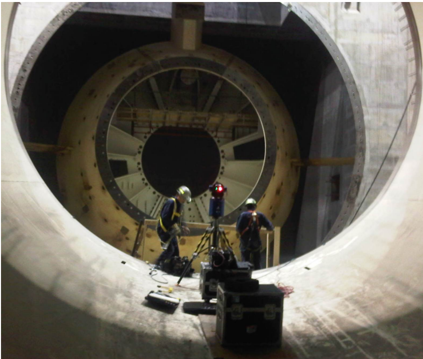
Figure 20: OASIS engineers align horizontal turbine components using laser tracker.
