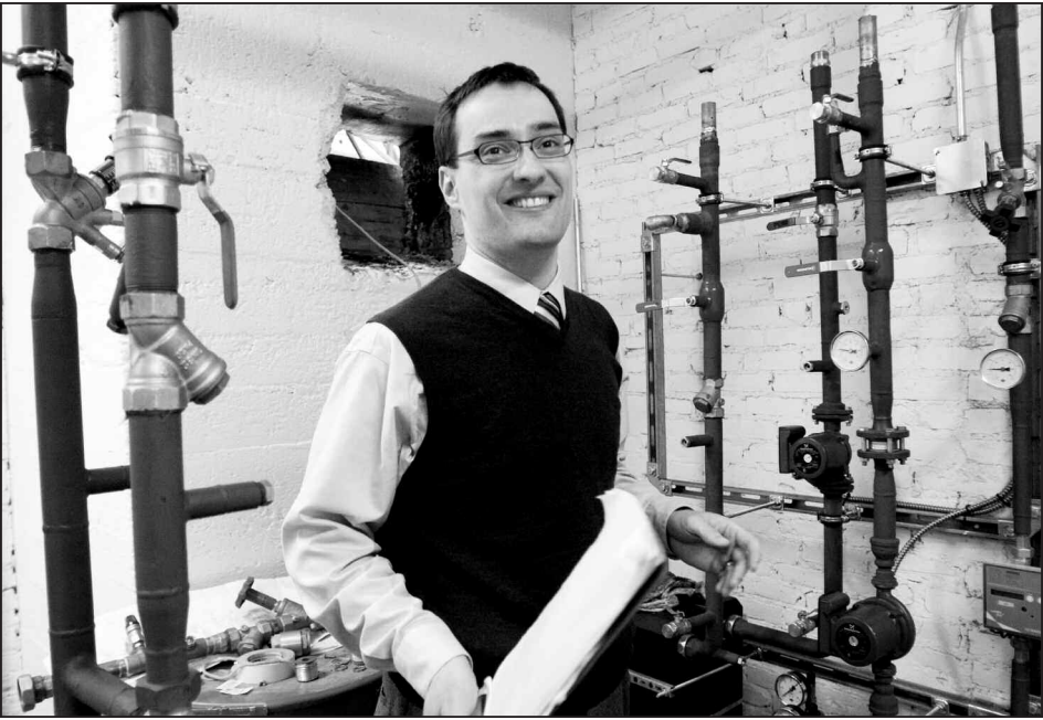
Bjorn Storz, program engineer at HRES, shows a coal chute and pumps where a glycol-water mix will circulate from solar panels to heat water.
