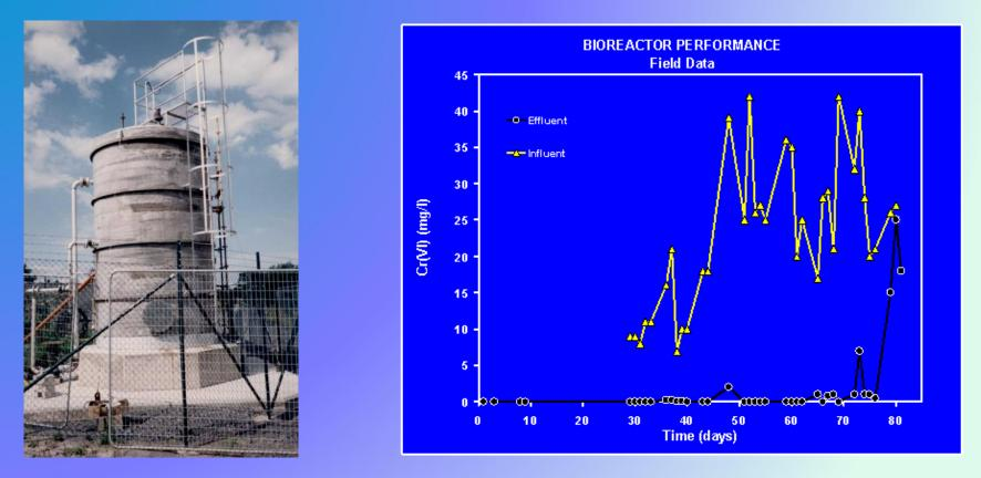
Our technology was incorporated into a 30,000 liter industrial bioreactor to remove Cr(VI) from waste leachate at a chromium steel factory in Sweden. Indigenous Cr(VI) reducing bacteria dominated the bioprocess that was fed acetate waste from a neighboring industry. The resulting Cr(III) precipitated inside the bioreactor as a hydroxide.
