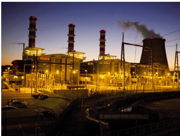
Fig. 1: View of a SCC5-4000F single shaft combined cycle power plant.
