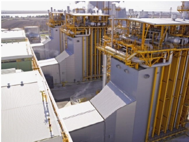
Fig. 5: Typical heat recovery steam generator.
