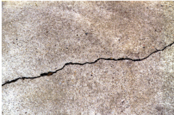
Figure 1.5 Fracture in concrete storage tank base.
