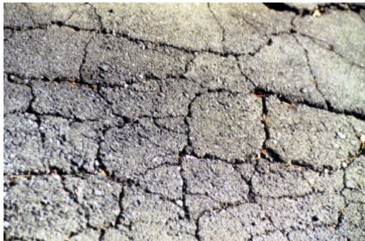
Figure 1.7 Fracture in asphalt liner.
