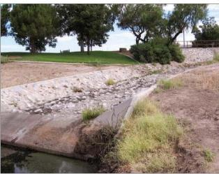
Much of the landscape design on the NMSU campus was created to manage storm runoff. From swales to cuts in curbs, it all serves a purpose – moving storm water away from buildings and to areas where it can absorb into the ground.
