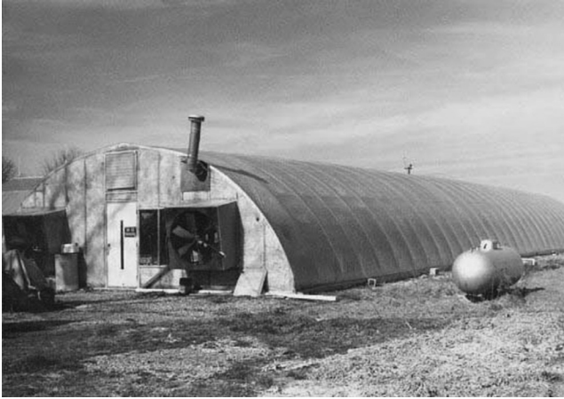
Figure 1.1 Quonset-style double-wall polyethylene-covered greenhouse (common design for most single-bay greenhouses primarily for use by an owner/grower operator).
