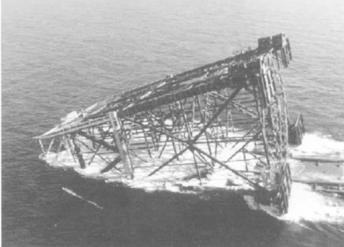
**Figure 14.27 Launching of a 4-Leg Jacket**
