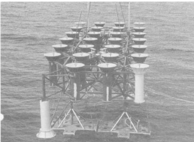
Figure 14.20 Subsea template lifting
