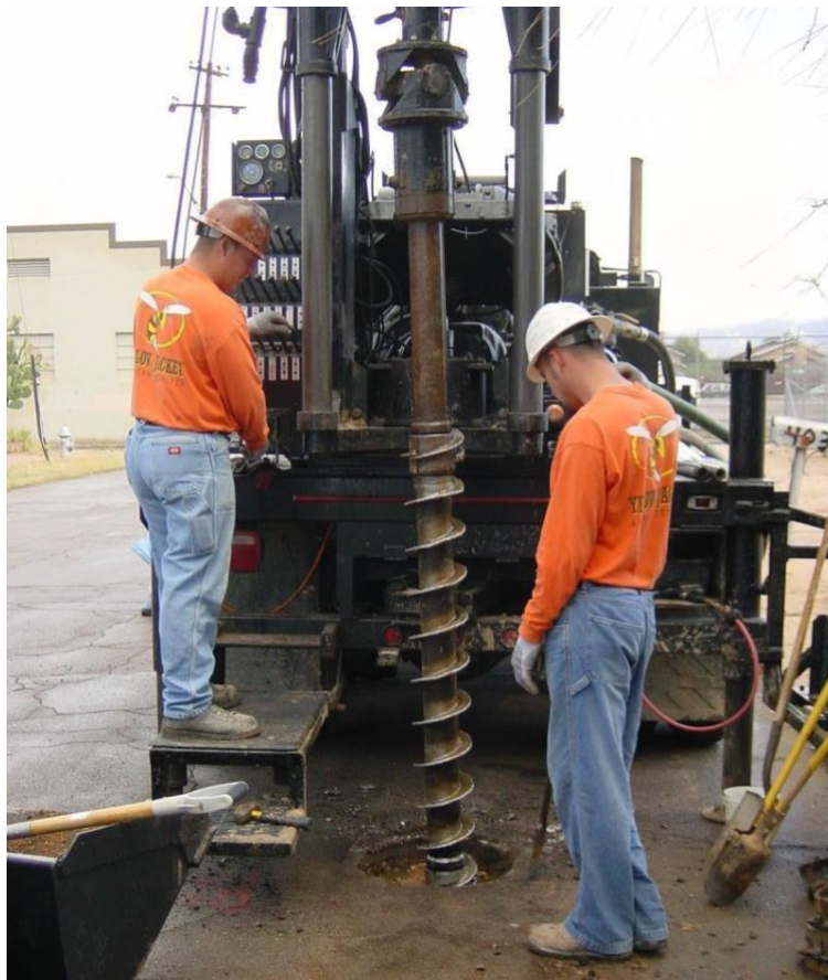
Groundwater monitoring well drilling and installation
