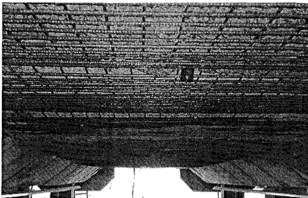
Fig. 19.11. All loose concrete has been removed from the slab. Photo courtesy of Betongfornyelse A/S, Norway
