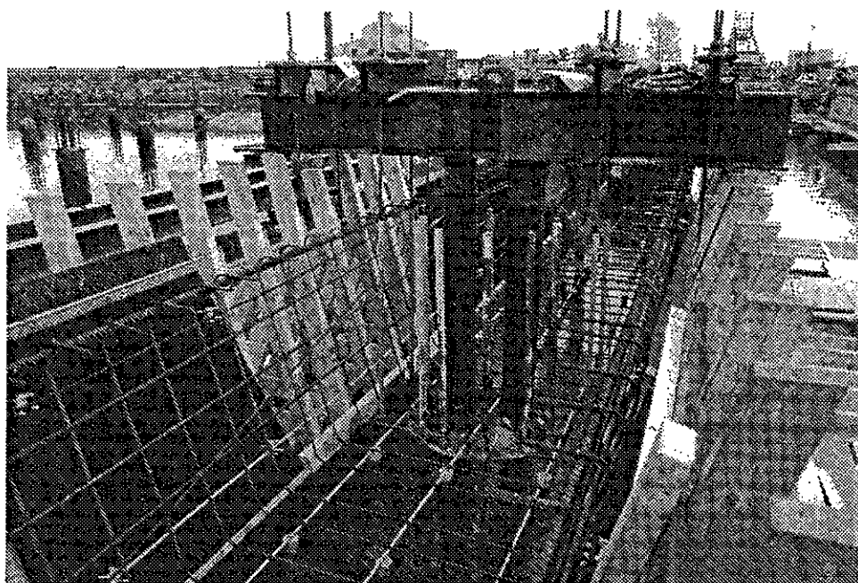
Fig. 11.34. The beam during the installation of the reinforcement with the beam formwork hanging from the column
