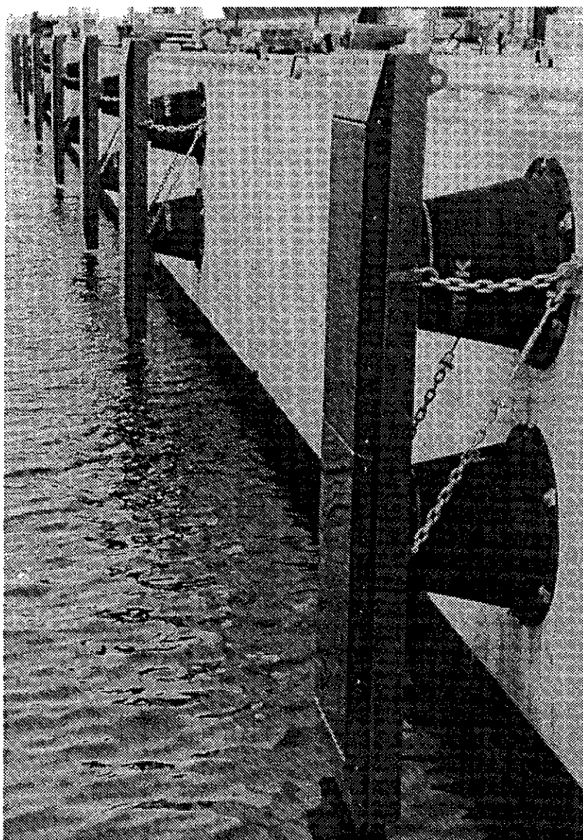
Fig. 14.40. Fentek super cone fender
