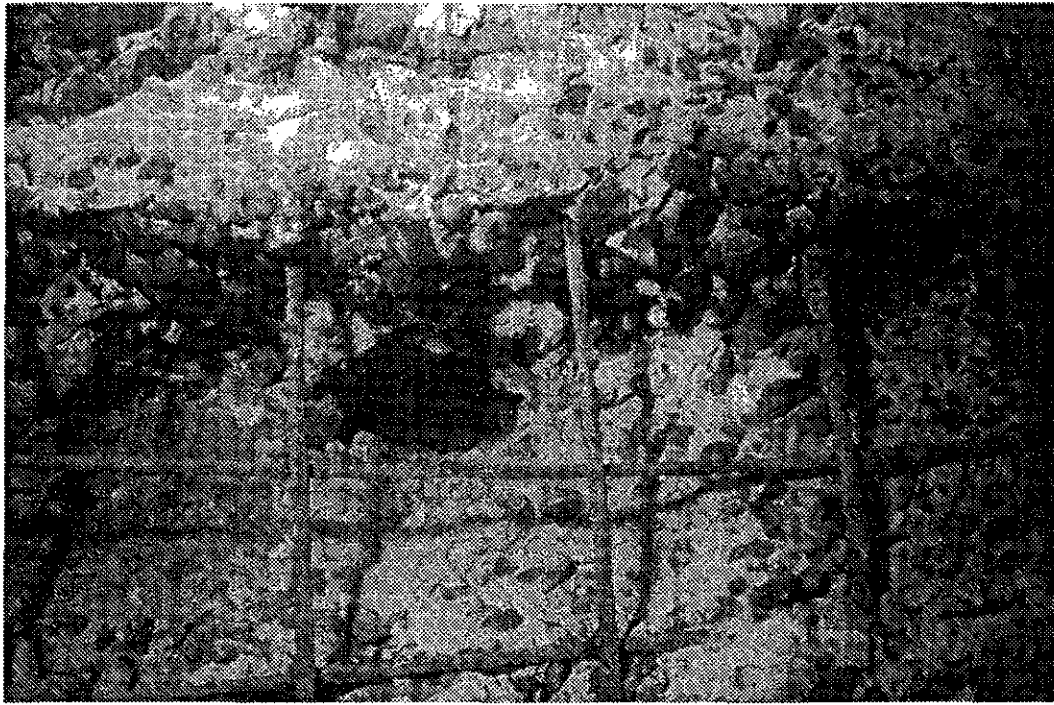
Fig. 19.1. Cleaned concrete surface before repair
