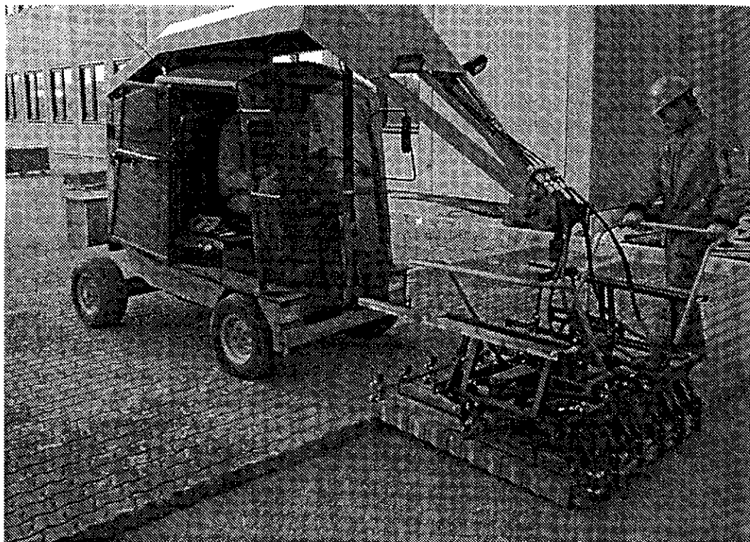
Fig. 12.13. Concrete pavers laid by machine
