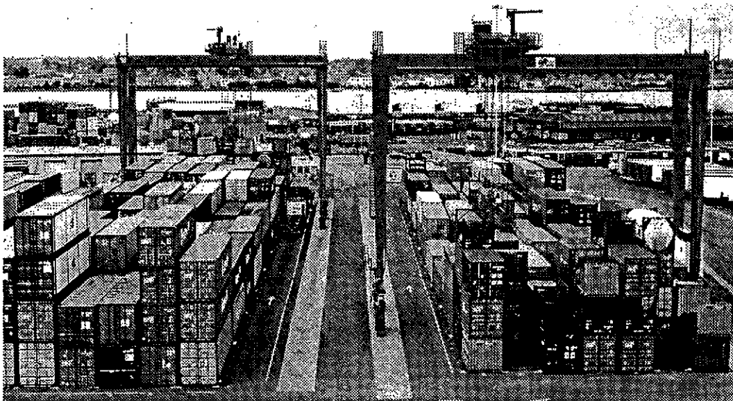
Fig. 13.18. Detail of RTG stacking 7 wide and 4 high
