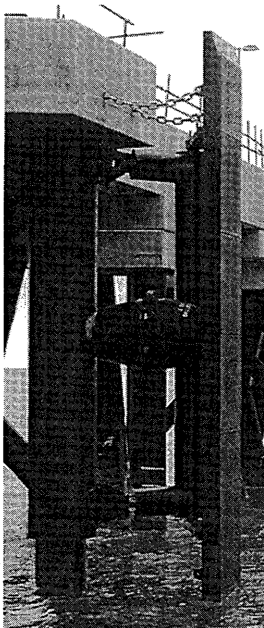
Fig. 14.29. Fentek parallel fender wall system with cone fenders
