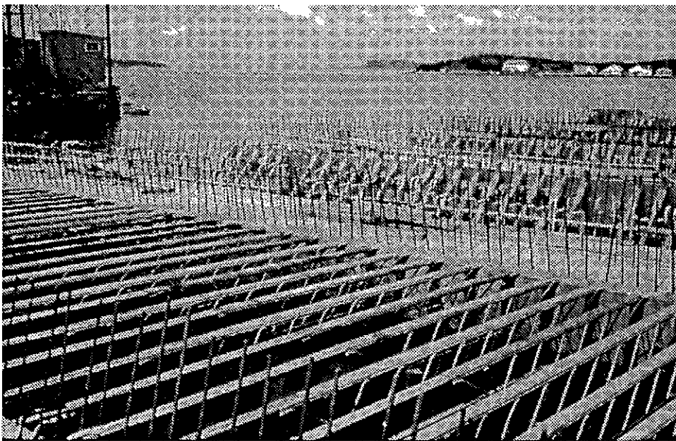
Fig. 11.33. Girders spanning between beams
