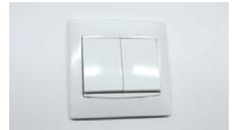
03 Install the cover plate of the switch
