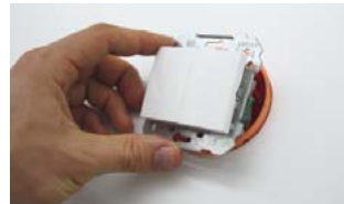
02 Install the switch over the switch coupler
