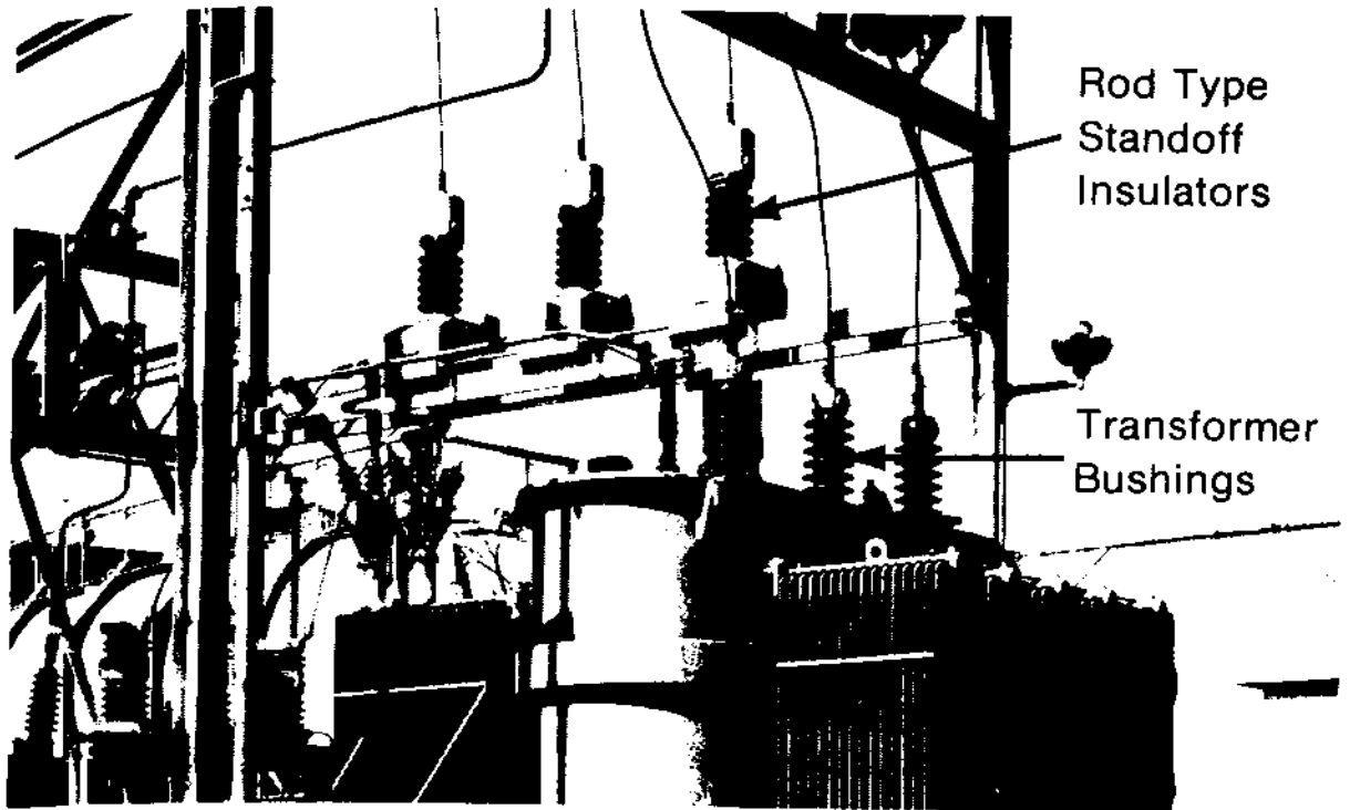
Figure 1.63 - A typical medium power transformer, highlighting transformer bushing and rod standoff insulator.
