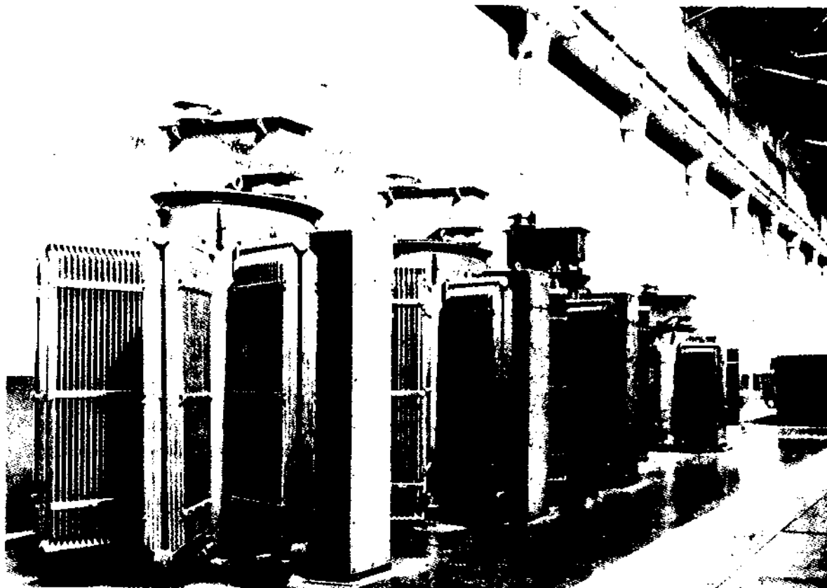
Figure 9.4 - A typical askarel transformer bank located inside a factory.
