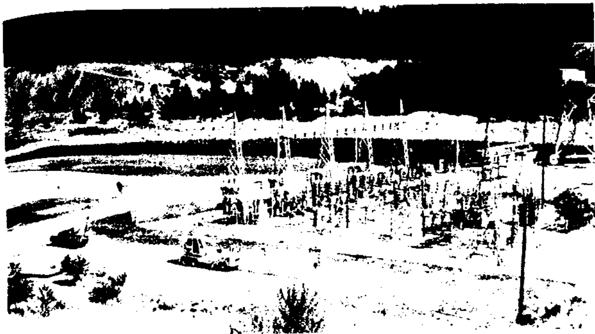
Figure 7.44 - On-site energized desludging of substation transformers has been performed for more than 30 years. Only recently has the electrical industry formally recognized that successful operation is being done; and done safely, resulting in many benefits—less downtime, lower labor costs and no transportation or rigging costs.
