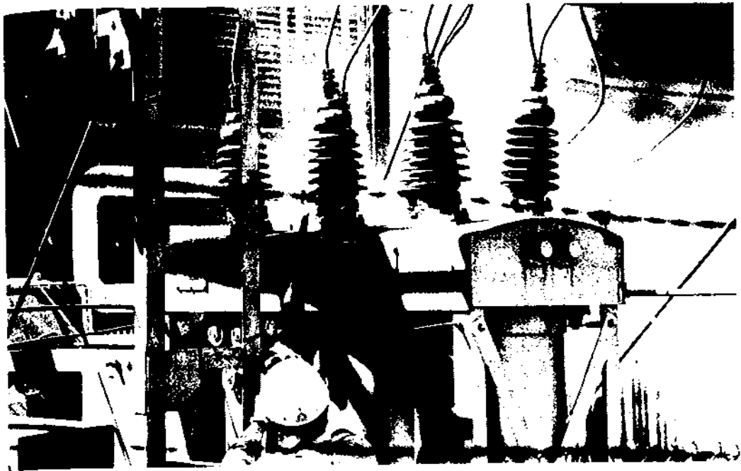
Figure 8.3 - A typical oil circuit breaker (OCB).
