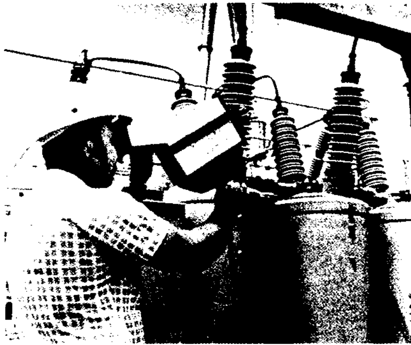
Figure 8.38 - Portable infrared scanner monitoring utility substations for electrical faults. (Courtesy of Xedar Corp.).
