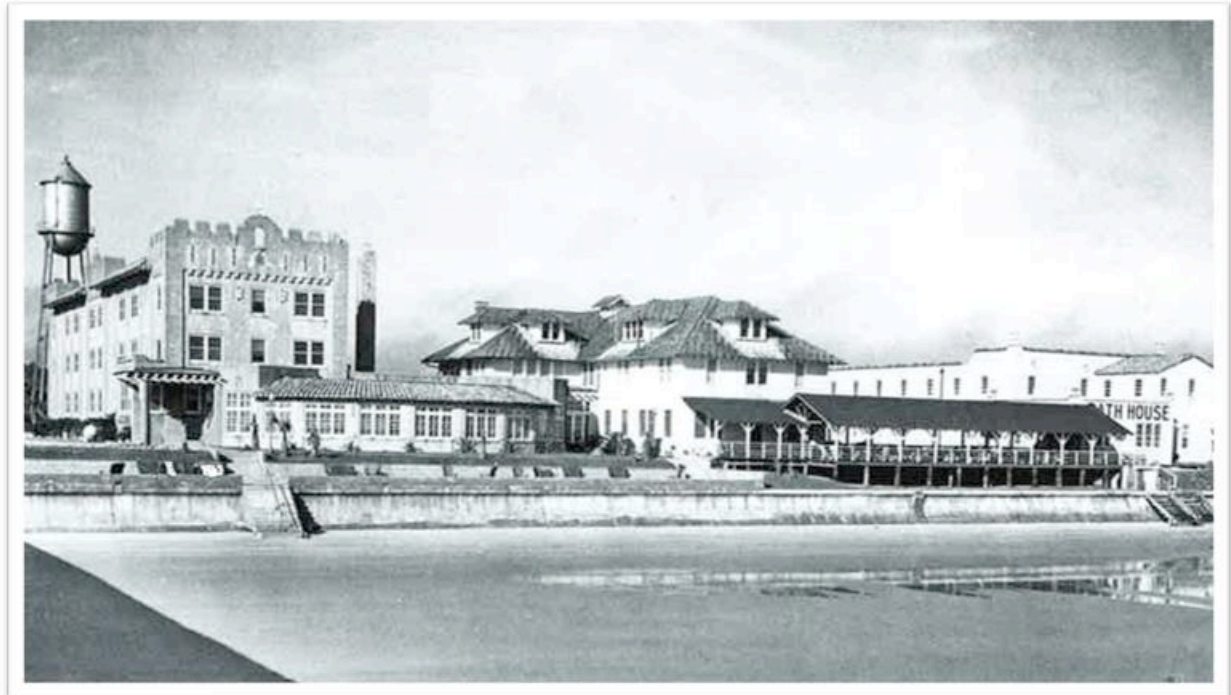
Figure D: Seawall construction along Atlantic Beach in the 1930's.
