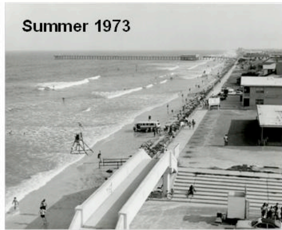
Figure E: Construction of the jetties at Mayport contributed to a lack of sediment supply for the downdrift (south) beach leading to a gradual lowering and contracting recreational beach. The problem was readily apparent by the early 1960's and continued until the initial nourishment project in 1978.
