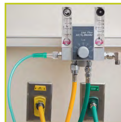
Figure 4.16. Flowmeter set to 10 L/min. Adjust blender to desired oxygen concentration.
