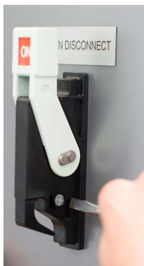
Figure 5-16 Example: Defeating with a screwdriver
