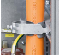
Figure 11-10 Cable clamp example
