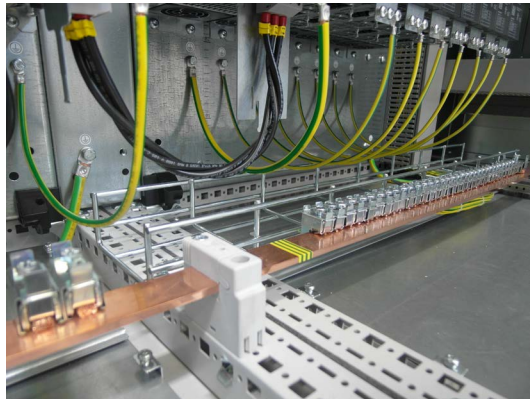
Figure 8-1 Grounding concept of an industrial control panel
