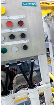
Figure 11-14 Conductors routed in raceways
