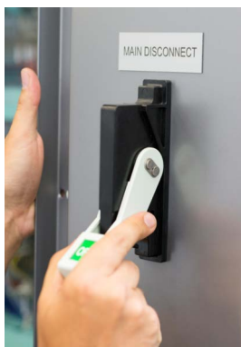
Figure 5-17 Example: Defeating without tools by actuating a lever on the reverse side of the door with the left hand.
