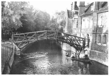
Fig. 1.2. The wooden bridge at Queens' College, a 1902 reconstruction of the original 'mathematical' bridge built in 1749 to William Etheridge's design.
