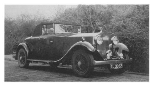
Fig. 27.6. A 1932 Rolls-Royce. Mounted on a separate steel chassis is an all-aluminium hand-beaten body by the famous coach building firm of James Mulliner. Any weight advantage due to the use of aluminium is totally outweighed by the poor weight-to-strength ratio of separate-chassis construction; but the bodywork remains immaculate after 48 years of continuous use!
