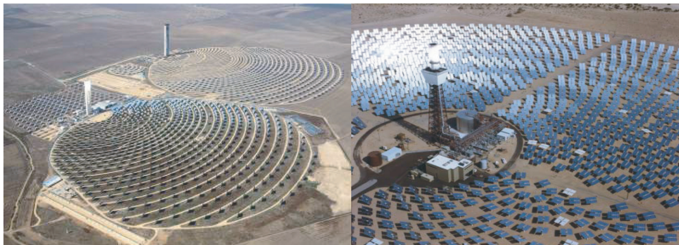
Figure 11.55 | PS10 and PS20 power towers in Spain (left) and a power tower solar thermal power plant in the California desert (right). Source: Left photo courtesy of Abengoa Solar.
