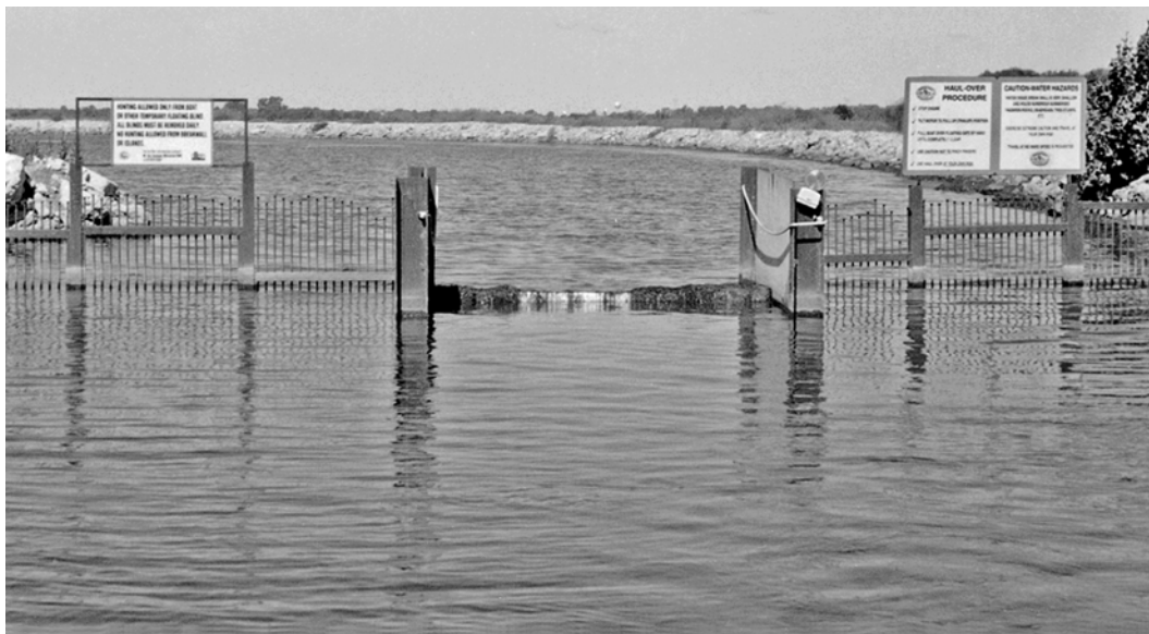
FIGURE 12.1 Carp exclusion gate at Terrell's Island restoration area. The center of the gate is spring loaded so that a boat pushes it down when entering or leaving the area.
