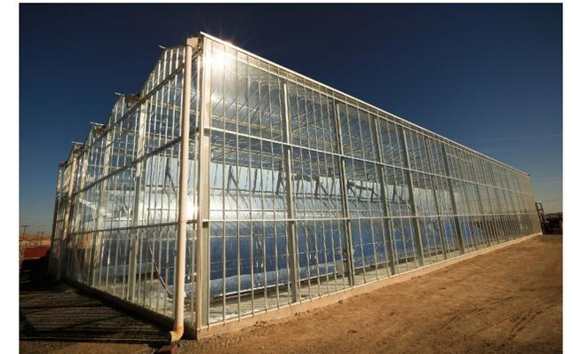
Solar Enhanced Oil recovery could displace 20% of NG use for EOR in CA: Kern County 21Z Solar Project (GlassPoint Solar)
