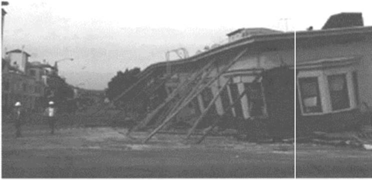
FIGURE 17.8 Collapsed wooden apartments with masonry veneer in the Marina District of San Francisco after the Loma Prieta earthquake. (Photo by the International Masonry Institute.)
