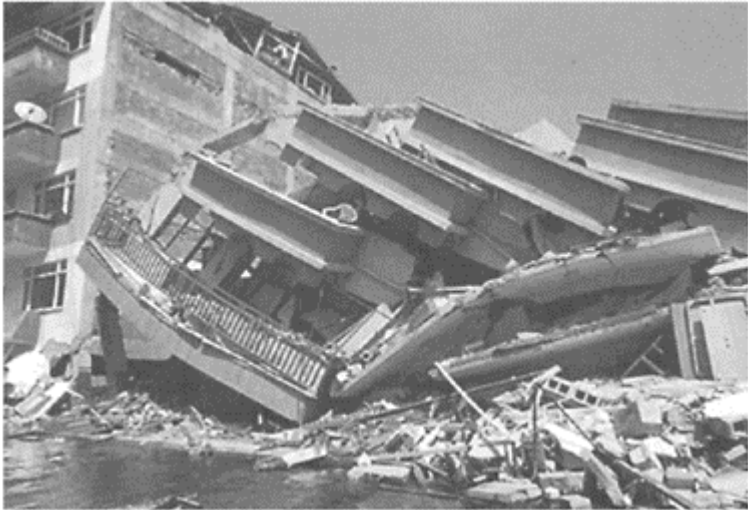
FIGURE 17.15 Damage to reinforced concrete frame with unreinforced masonry infill in Kocaeli earthquake. (Photo, EQE International.)
