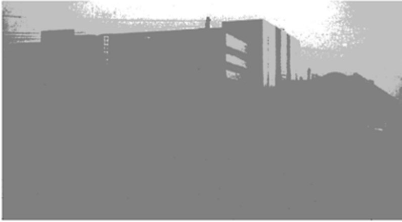
FIGURE 11.12 West Japan Postal Savings Computer Center: base-isolated building affected by the 1995 Kobe, Japan, earthquake.
