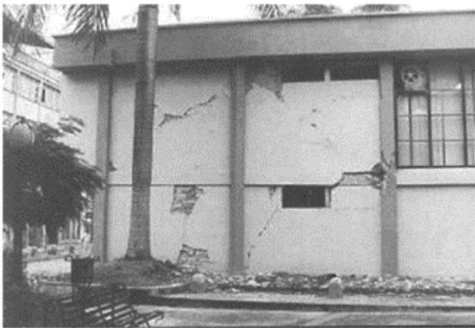
FIGURE 17.14 Damage to unreinforced masonry
