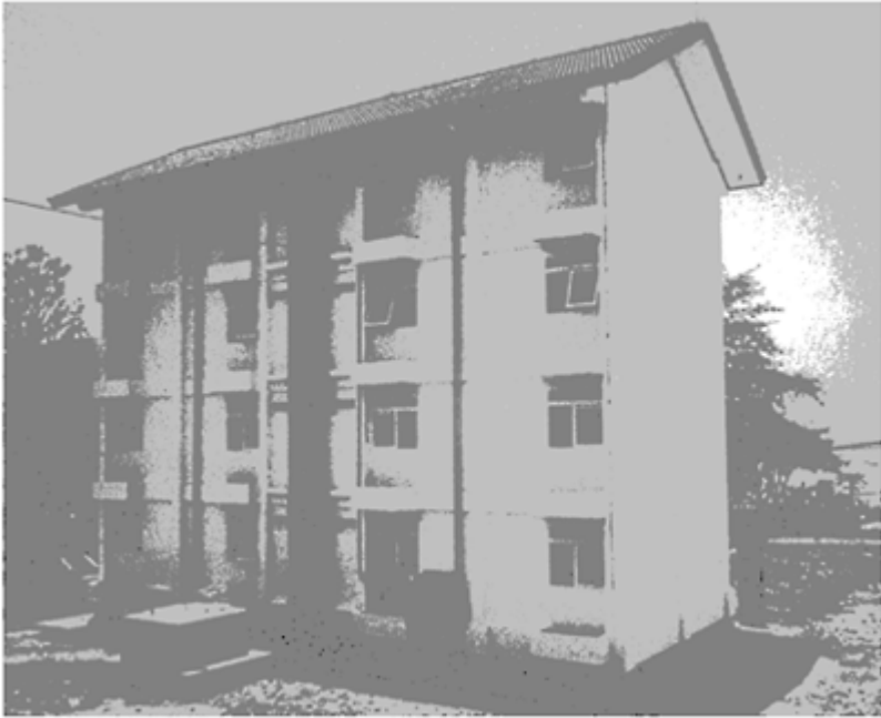
FIGURE 11.3 UNIDO demonstration base-isolated building in Indonesia.
