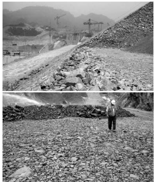
Fig. 1. Typical rockfills used in dam construction
