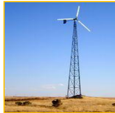
Figure 16: A small wind electric system called the Jacobs 20-kilowatt turbine can provide electricity for a variety of electrical needs from home heating and lighting to water pumping for livestock. Source: NREL.gov
