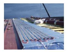
Figure 40: Dawn Solar Hot Water Heater Coils (Dawn Solar)
